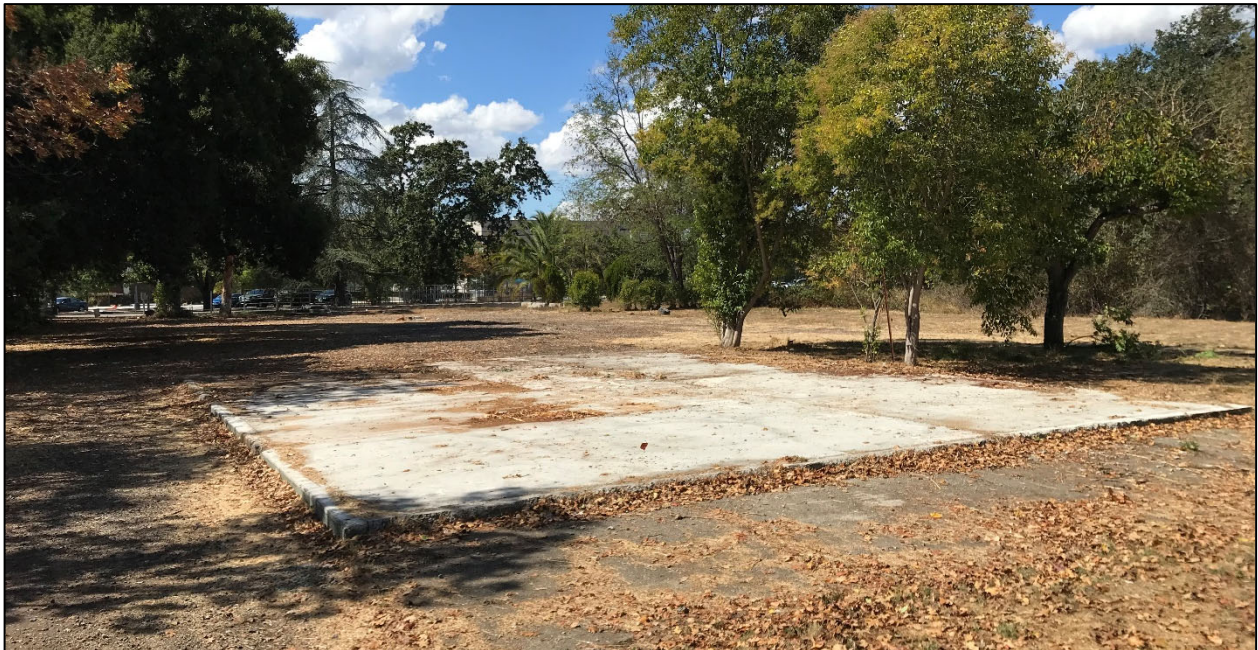
Photograph 2. Photograph depicting remnant concrete pad within the Project Area.
