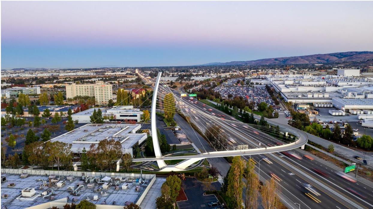
**Figure 12-6 Iconic Cable-stay Overcrossing Bridge with Horizontal Arch over I-880**
