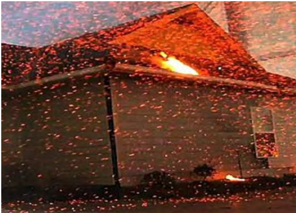
Photo 7 – Ember Shower. Roofs that are not Class A fire rated, vents that are not ember resistant, and combustible material that is located adjacent to a home can all contribute to the loss of a structure. Note the fire on the roof and the landscaping adjacent to the structure. Photo credit to the Insurance Institute for Business & Home Safety.
