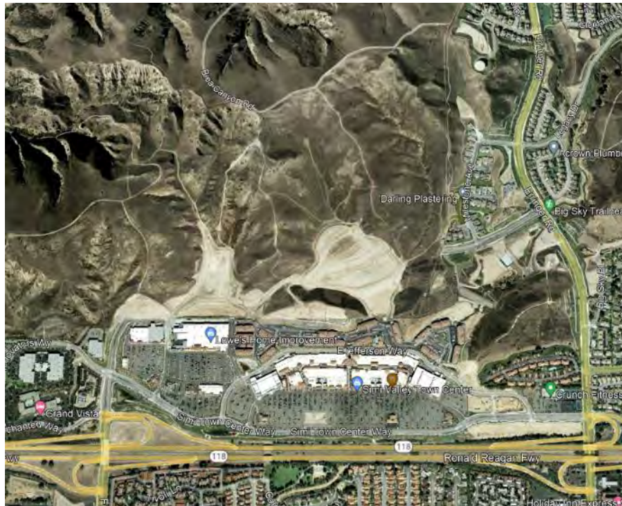
Photo 2 - Aerial Photo of Project Site, September 2007. At the time, the previous owners had graded the site in anticipation of construction.
