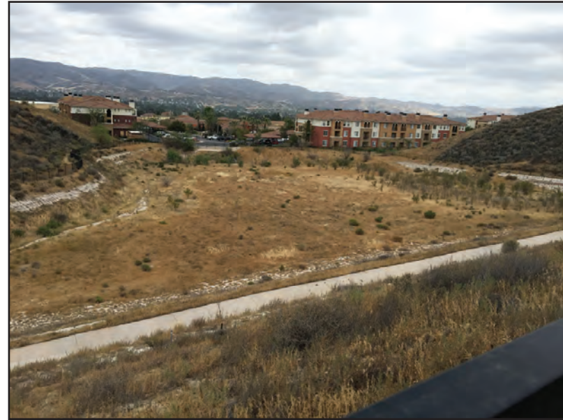
Photo 3B – View to the south of Debris Basin 2.
