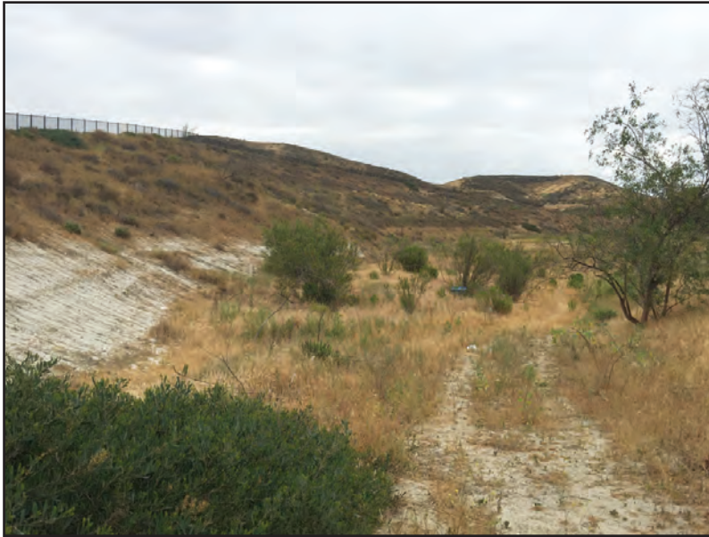
Photo 3A – View to the northeast of Debris Basin 1.
