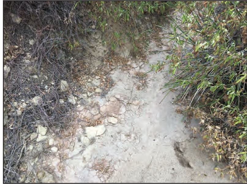
Photo 4B – View to the northwest of surface cracks within Drainage 9 in an area previously delineated as flowing water.
