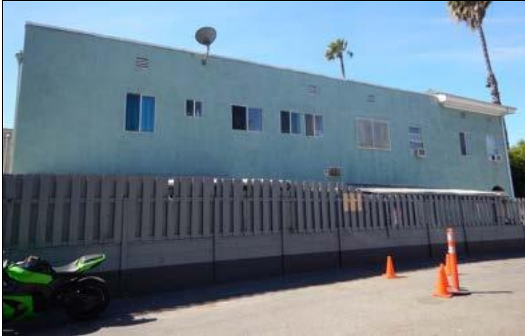
Figure 8. 812-814 South Mariposa Avenue., north elevation
