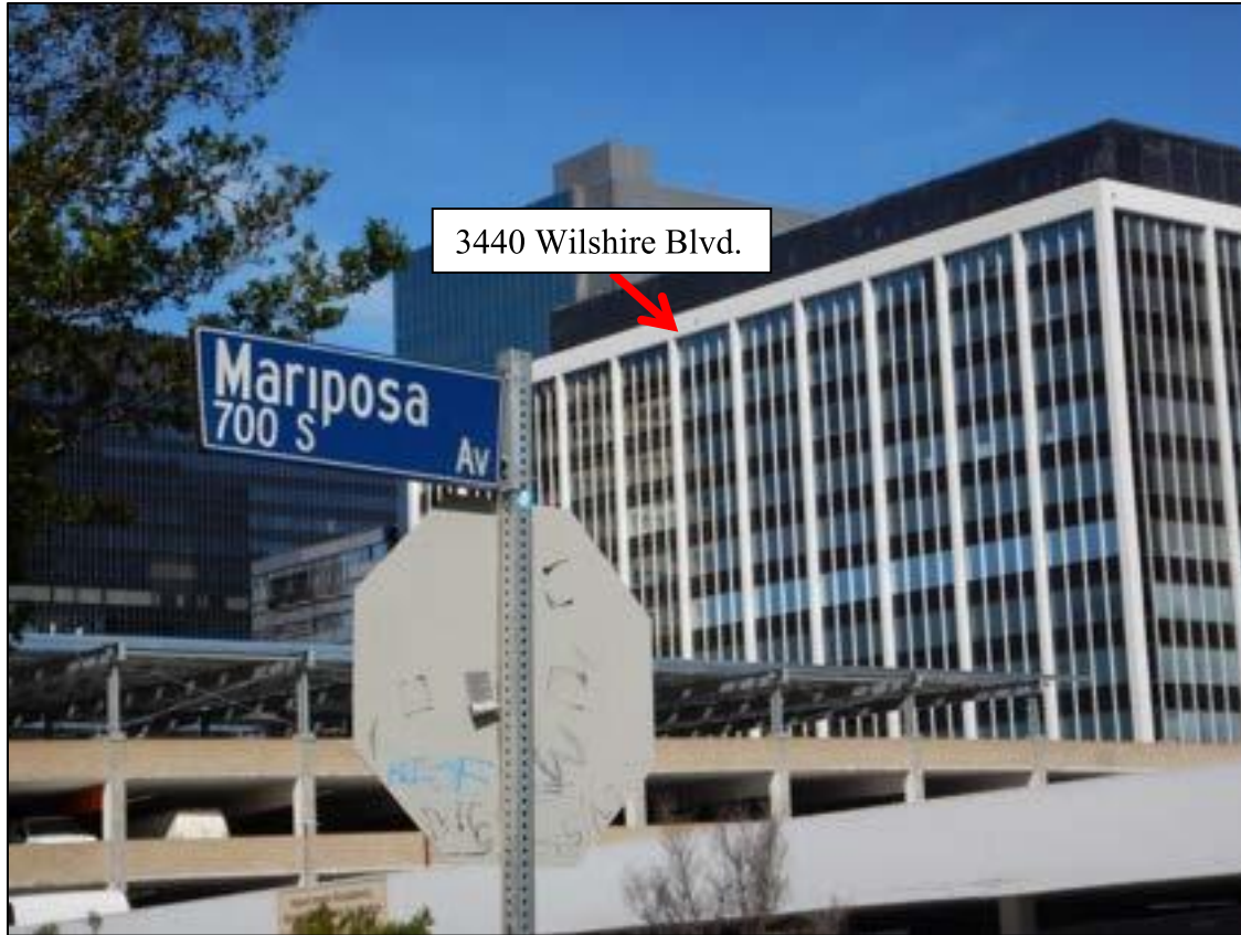
Figure 17. Corner of South Mariposa Avenue and 7 th street
