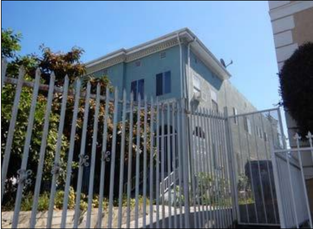
Figure 10. 812-814 South Mariposa Avenue., west (left) and south (right) elevations
