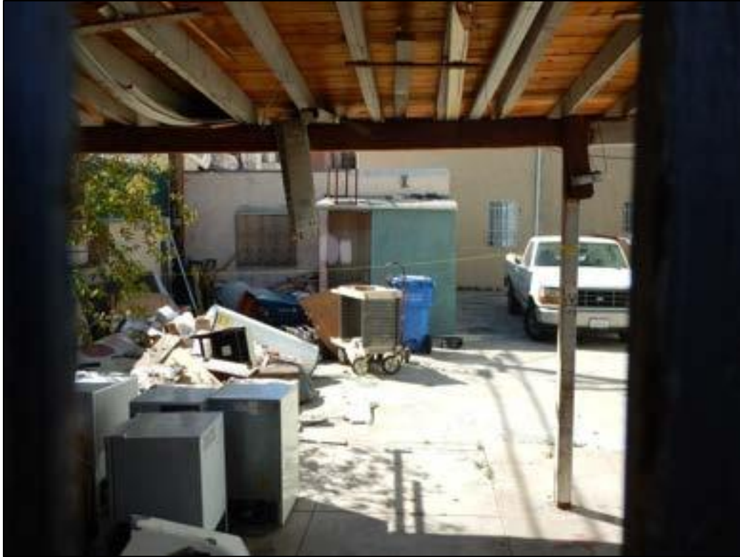
Figure 12. 812-814 South Mariposa Avenue., detached garage, north elevation Photo taken to show interior of wood-plank overhang
