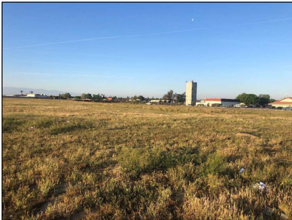
Project overview. View to southwest.
