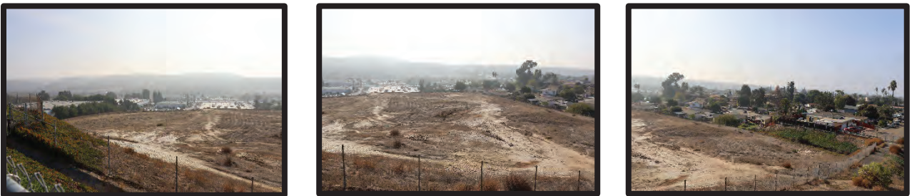
Figure 17 - Photos Looking to the South Across the Project Site
