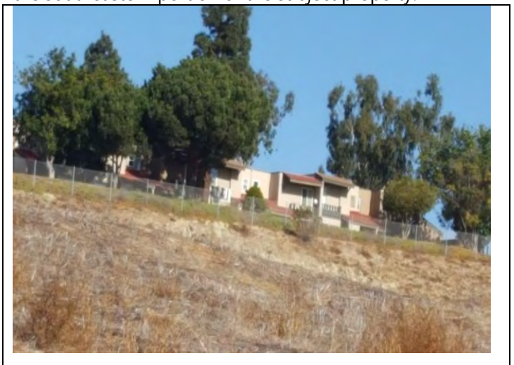
18. North-adjacent residential condominium complex beyond the northern portion of the subject property.
