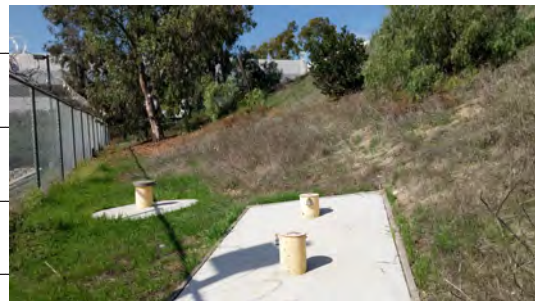
Waste cell Program Wells MW-02, MW-03, & MW-08
