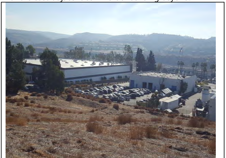
16. The southeast- and south-adjacent properties beyond the southeastern portion of the subject property.
