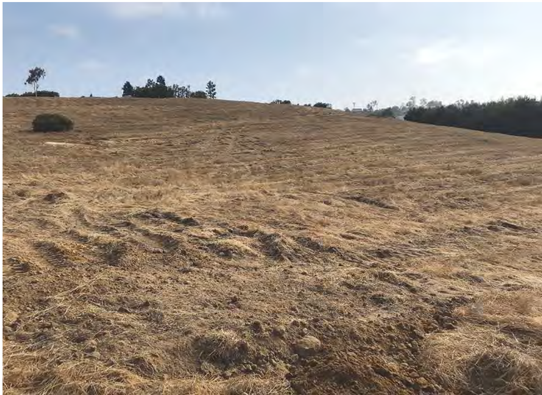
2) View of the Site looking northeast.
