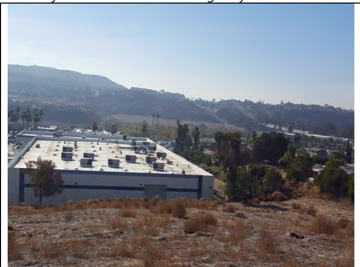
11. The southwestern portion of the subject property with one of two south-adjacent buildings beyond.
