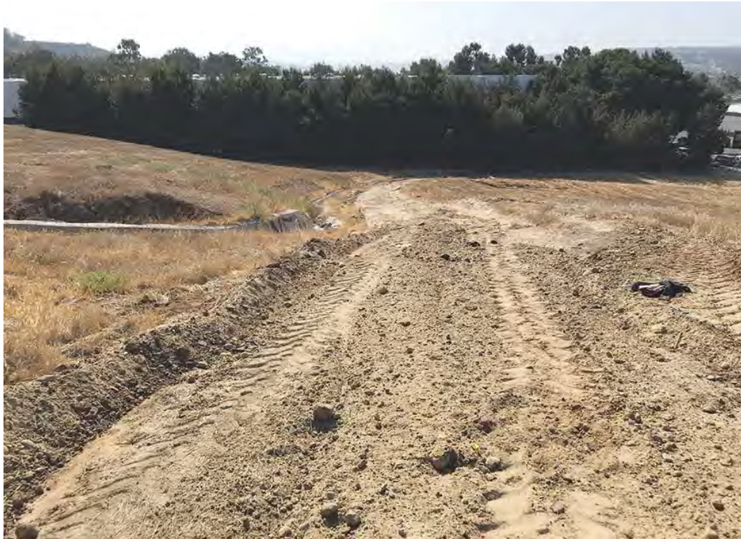
2) View of the roadway and concrete drainage in the east portion of the Site.
