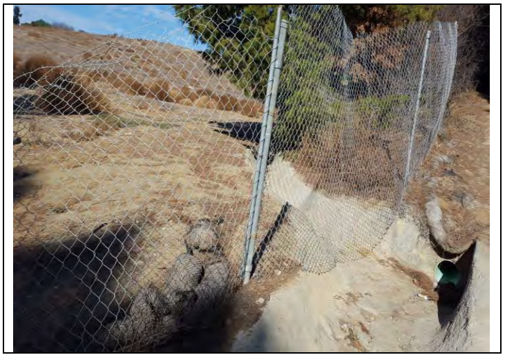
2. The southeastern portion of concrete stormwater channels throughout the subject property.
