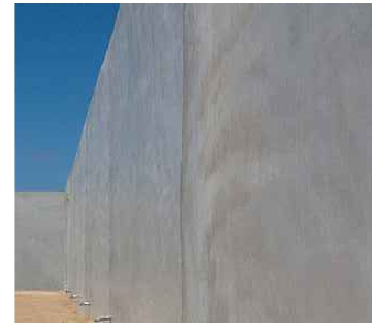
SOIL NAIL WALL SMOOTH TROWEL FINISH COLOR TBD
