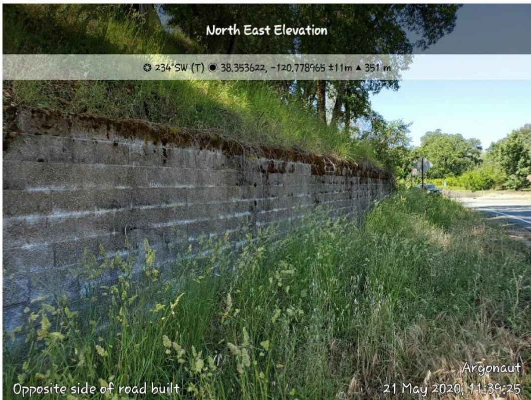
Figure 10. Retaining wall built across Sutter Street
