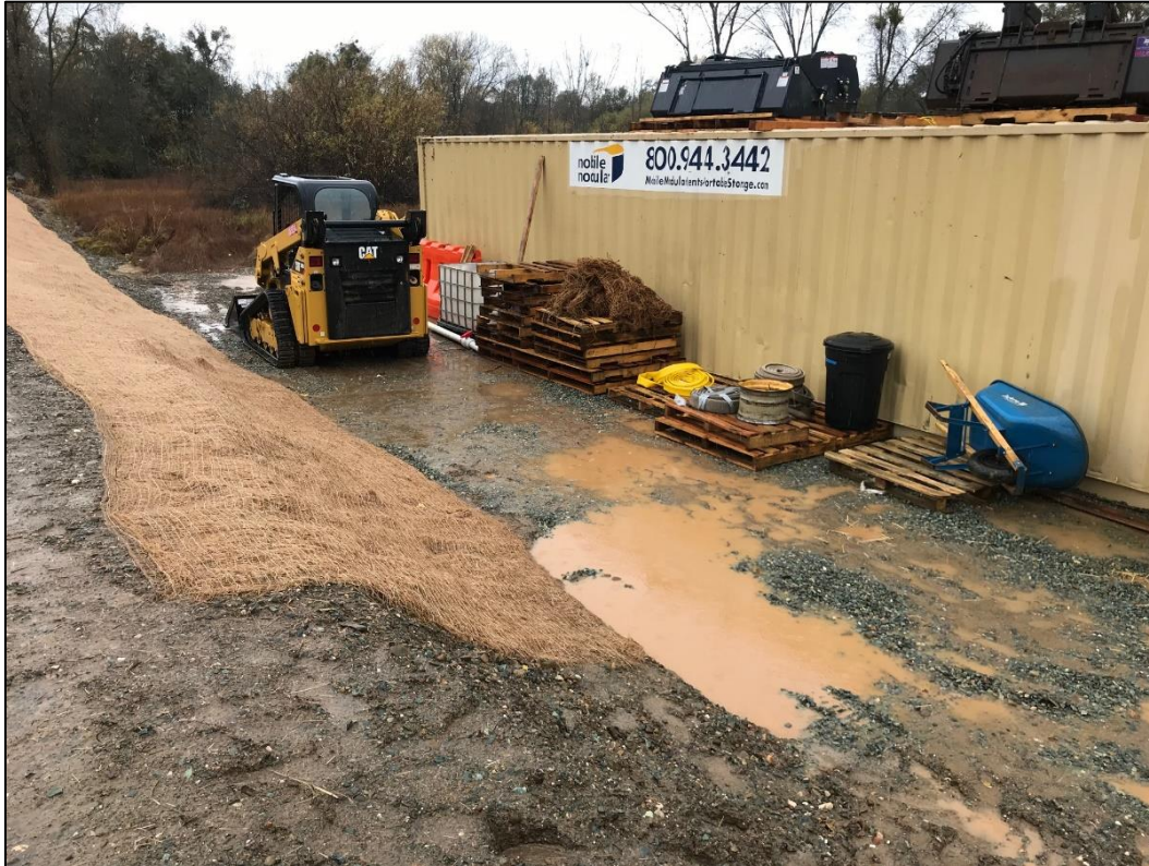
Figure 14. Prior use of staging area
