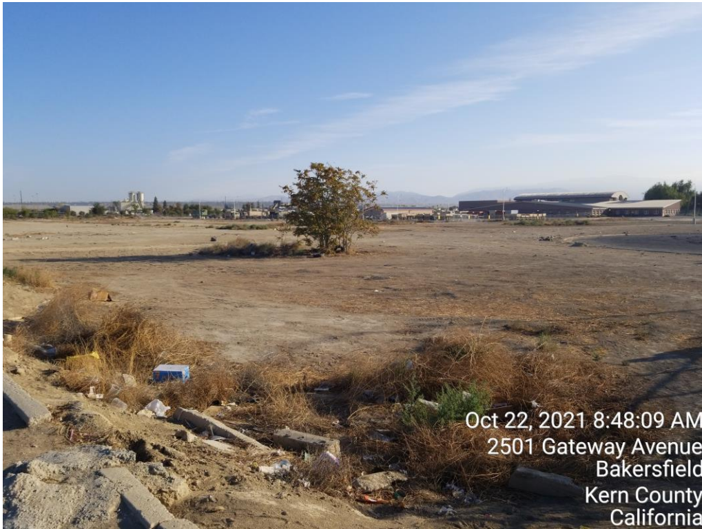
Photo B-3: Photograph of the project site taken at the southwest corner facing northeast
