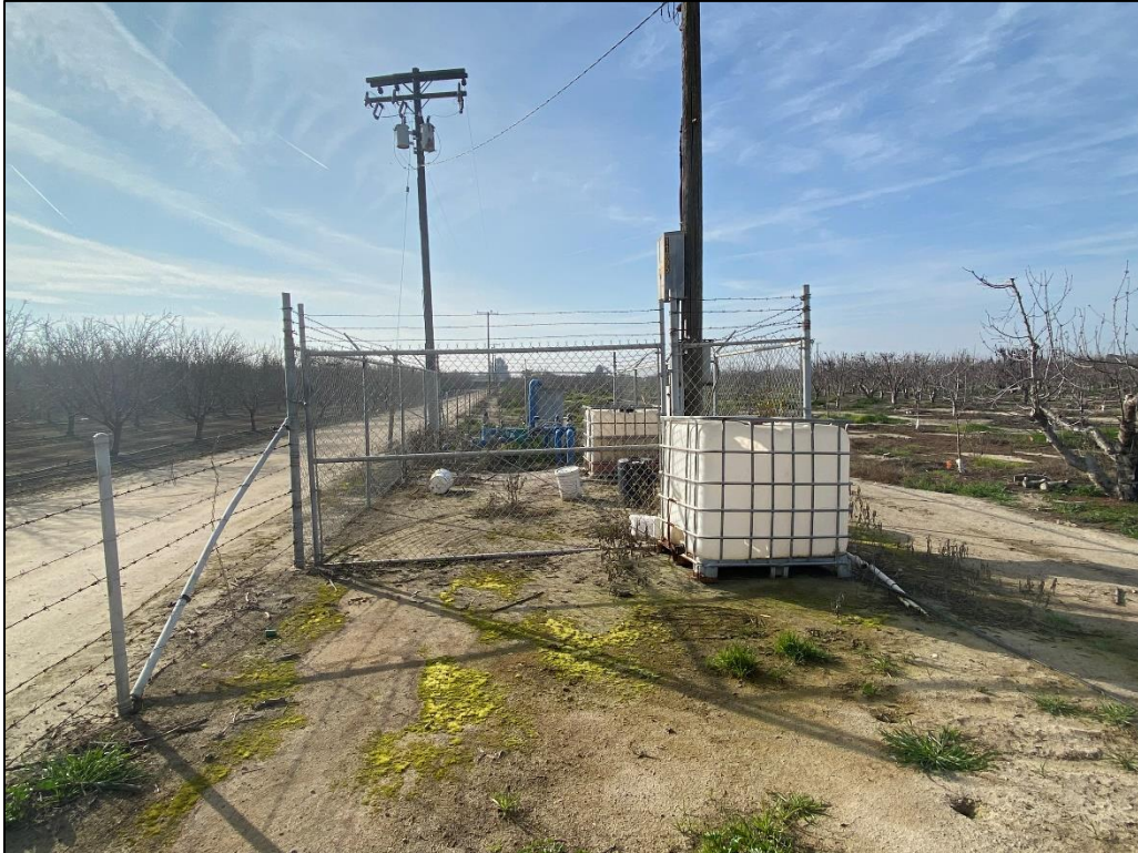
Figure 4-2 Northeastern portion of Project site, facing south. Irrigation pump in background.
