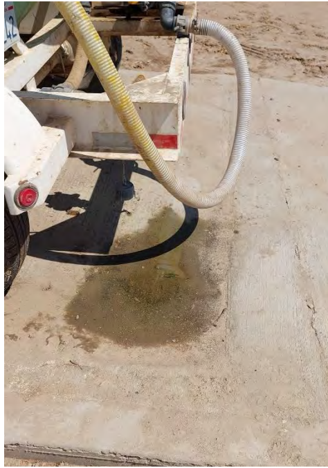
Photograph 7: Observed leakage on platform of AST mentioned in Photograph 6.
