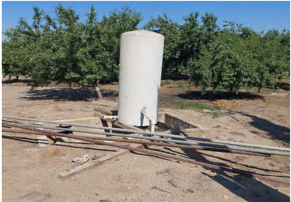
Photograph 2: Abandoned tank observed looking northwest of Road 89. Next to power box in Photo 1.
