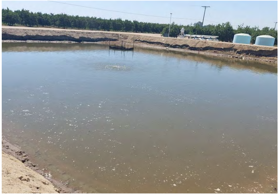
Photograph 5: View of pond, looking towards the southeast, located west of Road 89.
