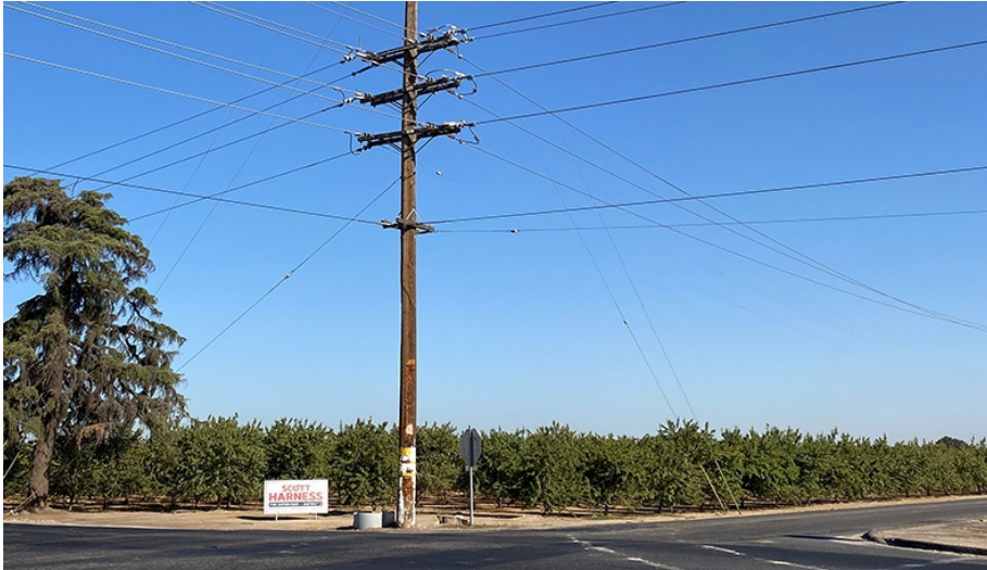
Photograph 1: View from the southeast corner of the project site at Shirk Street and Riggin Avenue; facing northwest.
