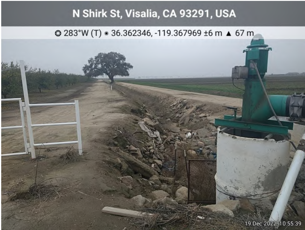
Photo 7. View of Modoc Ditch from Road 92, facing west.
