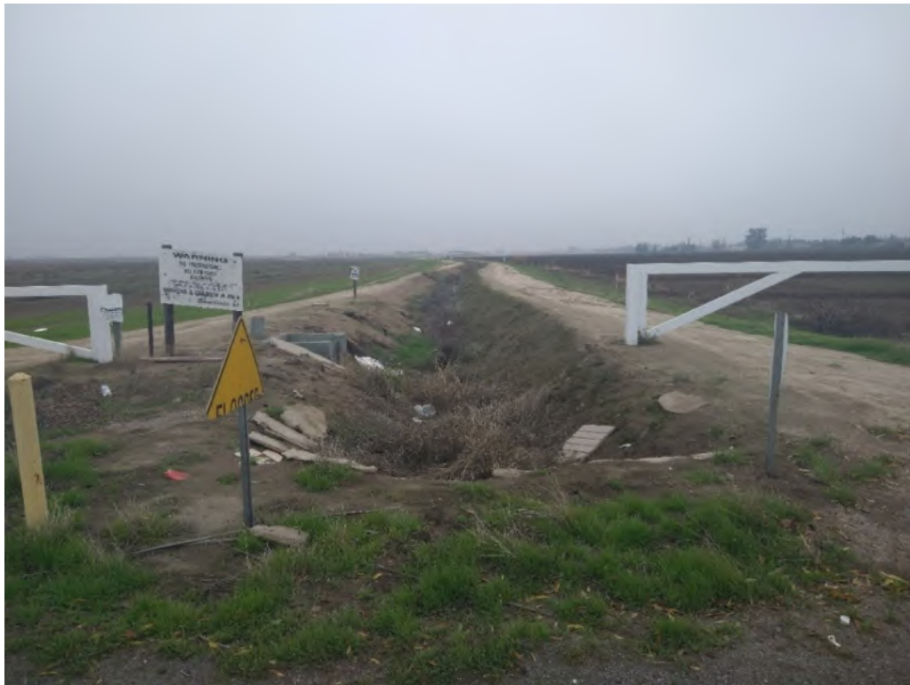
Photo 4. View of Wutchumna Ditch from Road 92, facing east.
