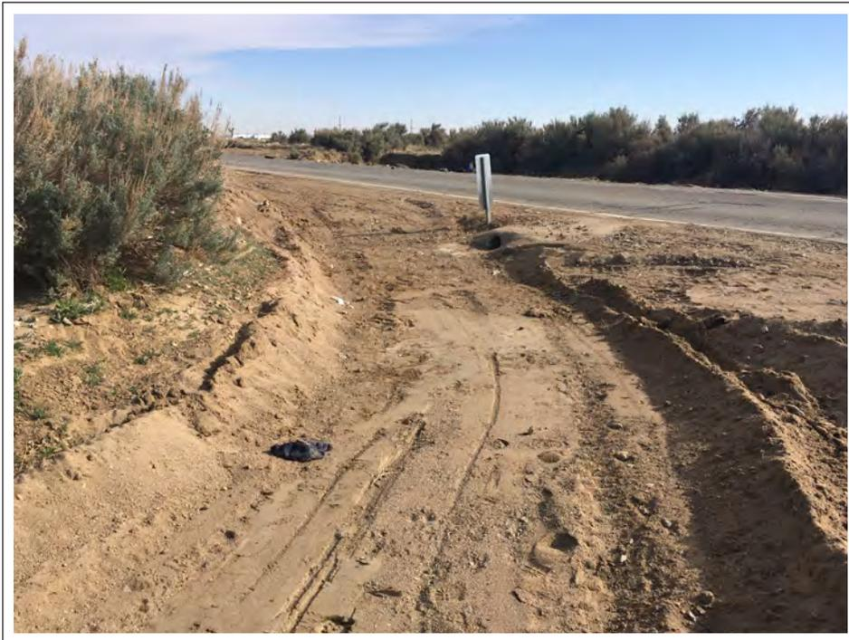
Photo Location 6, facing downstream. March 17, 2022. View of conditions where stream channel flows toward 8th Street along eastern site boundary. Note that road shoulder is graded to allow water to flow off road into channel. Small culvert is evident that allows water to drain eastward under 8th Street.
