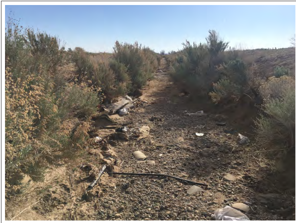
Photo Location 2, facing downstream. March 17, 2022. View of general conditions in stream channel.
