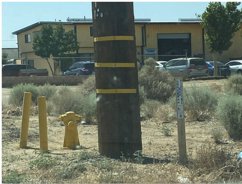
Looking west from south edge of site along Avenue M at utilities (hydrant, power pole, and gas pipeline locator) and transmission/auto shop west of 5 th Street East
