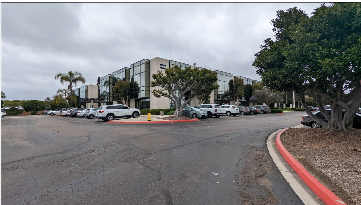
Existing structure at 6540 Lusk Blvd, view to the northwest. 5/27/2022.
