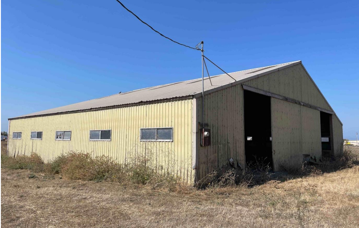
Photograph 3. Barn structure in northwest area of proposed annexation area .
