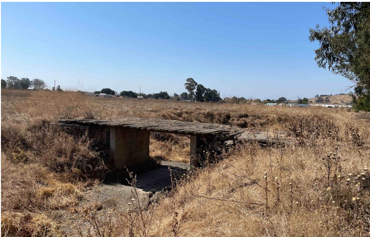
Photograph 4. Bridge crossing North Slough.
