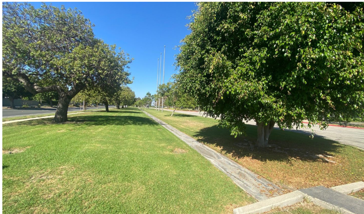
Photograph 3: View of shallow concrete ditch looking along substantial length from inlet that comprises terminus of shallow concrete ditch. Note turf on both sides of ditch.
