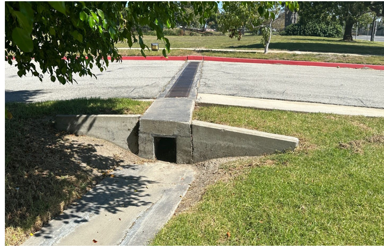
Photograph 6: View of shallow clean concrete ditch looking east at inlet.
