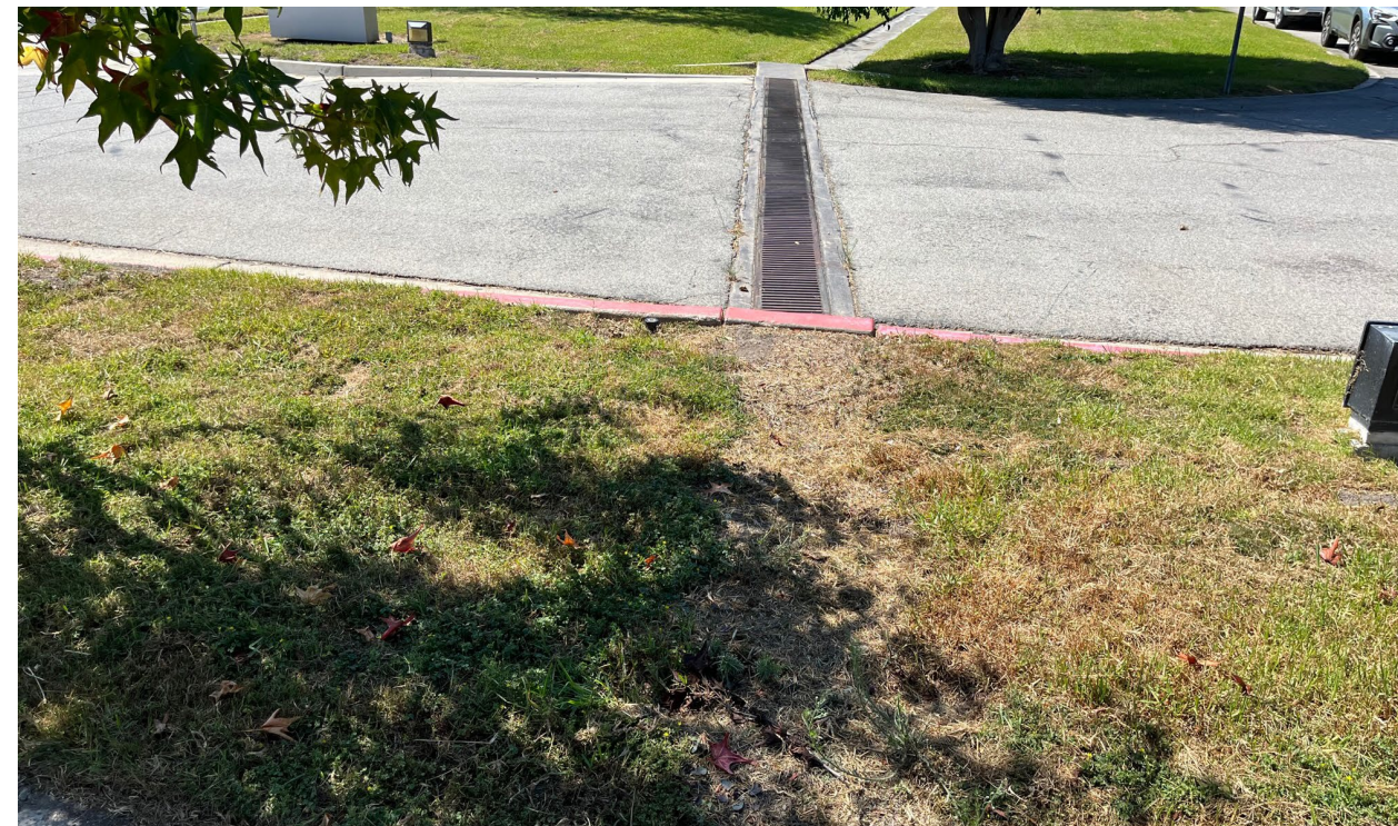
Photograph 8: View of turf at end of pipe which is currently completely plugged by sediment.
