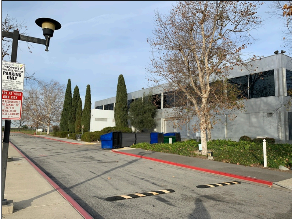
Photo 6: View of the west portion of the subject structure looking northeast.
