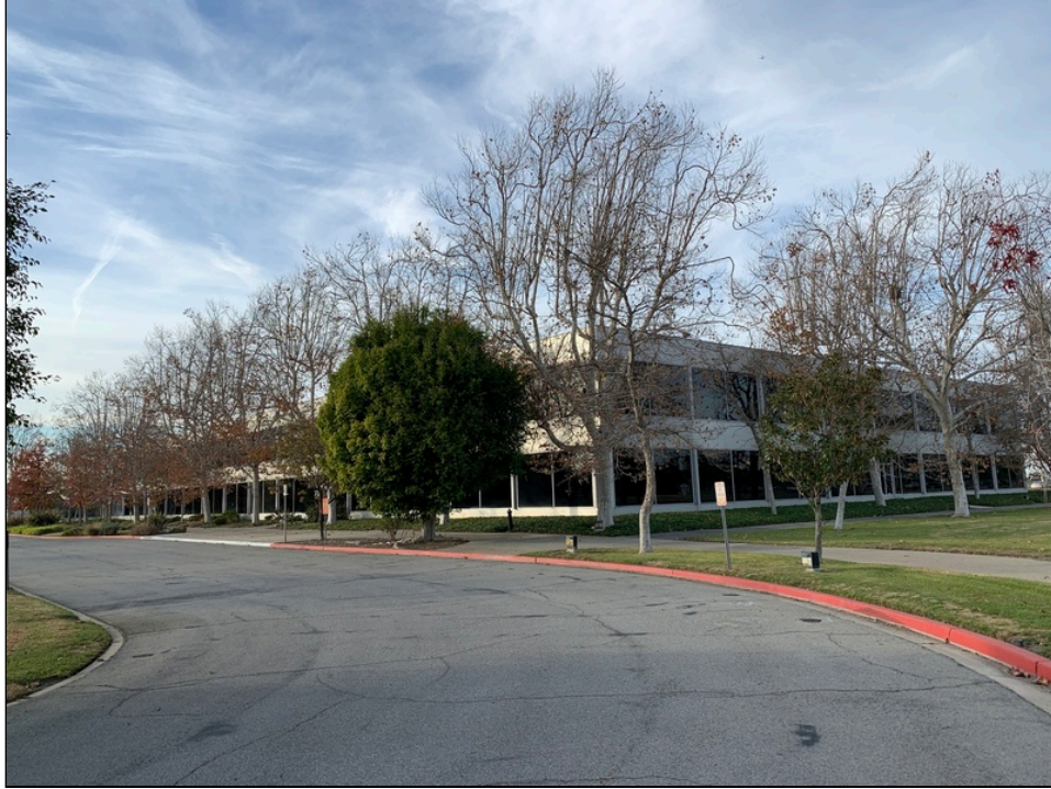
Photo 3: View of the southeast portion of the subject structure looking northwest.
