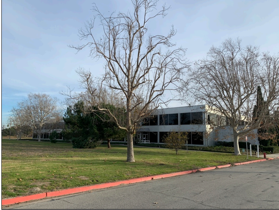
Photo 5: View of the northwest portion of the subject structure looking southeast.
