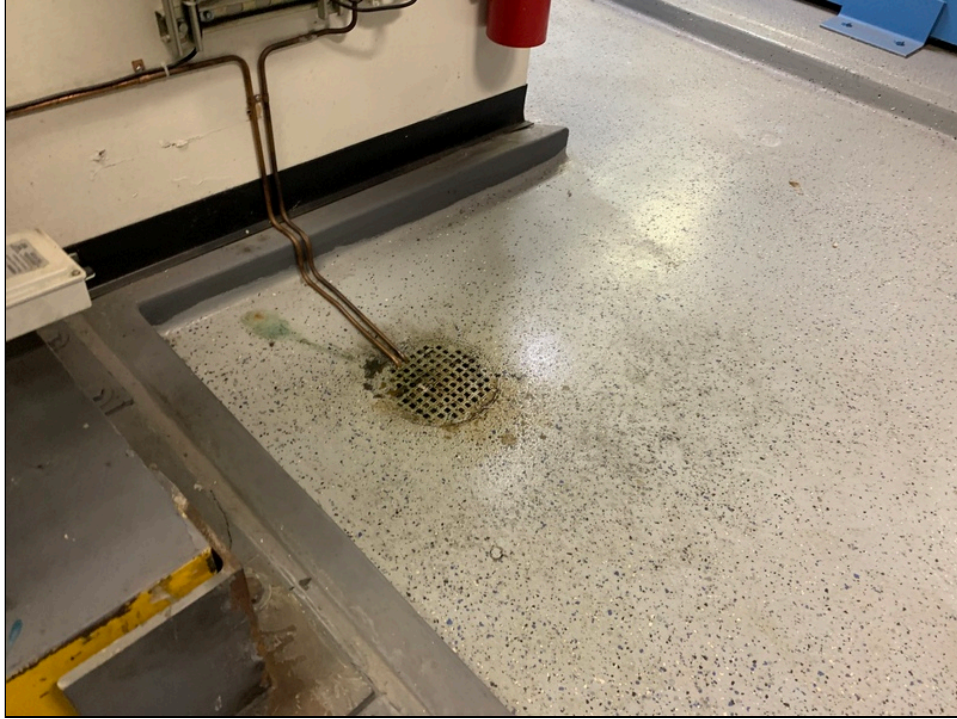
Photo 41: View of drain within the chiller room.
