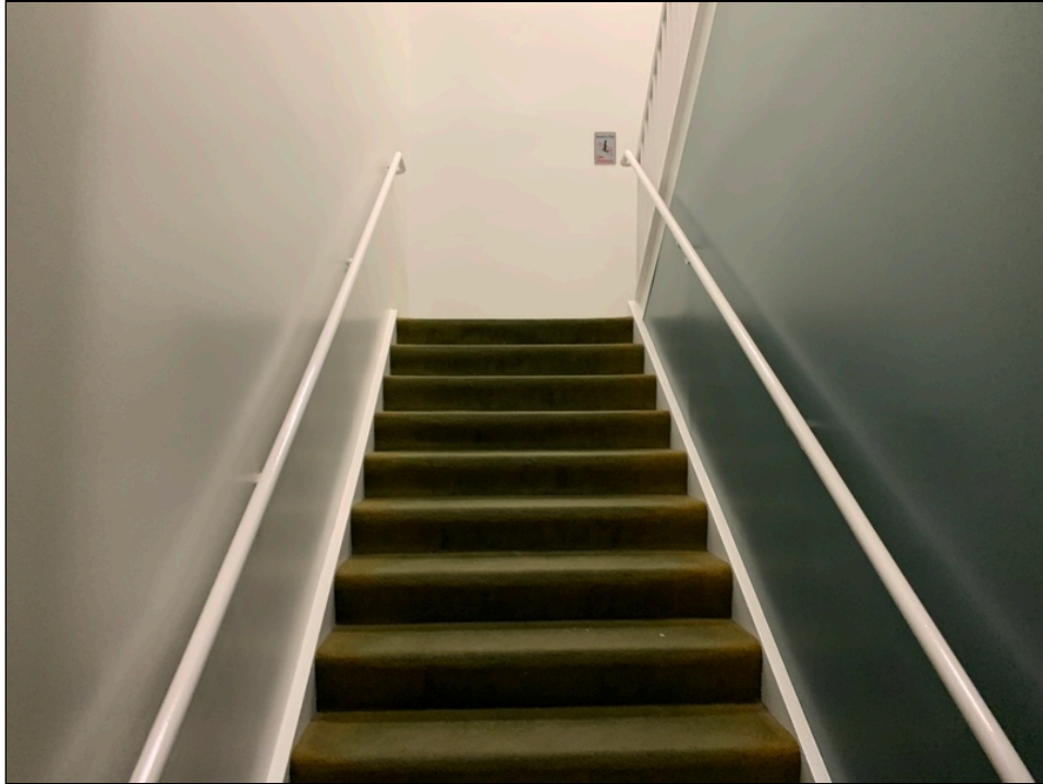
Photo 32: Representative view of stairs.
