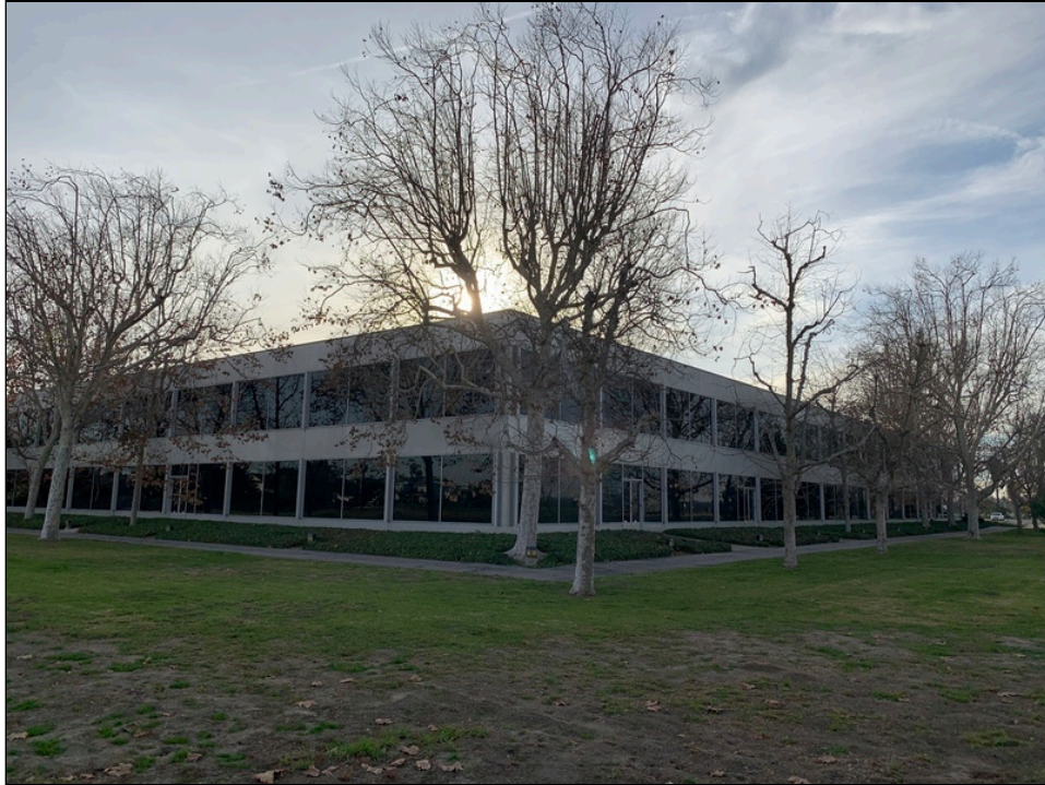
Photo 4: View of the northeast portion of the subject structure looking southwest.
