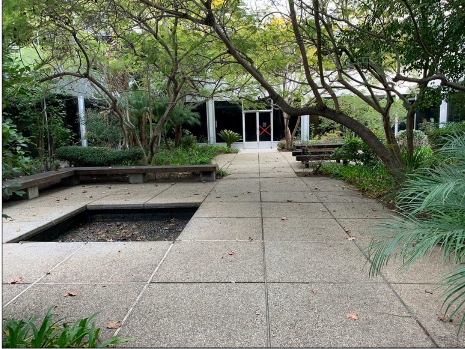
Photo 7: View of the courtyard on the central portion of the subject structure.
