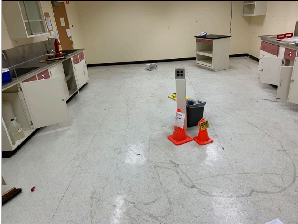
Photo 43: View of former laboratory.
