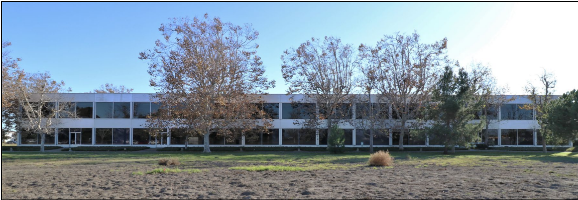
North elevation, view south (11/18/22).
