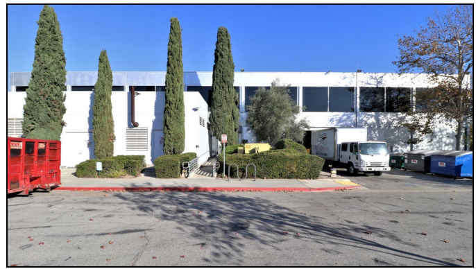
West elevation with addition on the left side of the photograph, view east (11/18/22).
