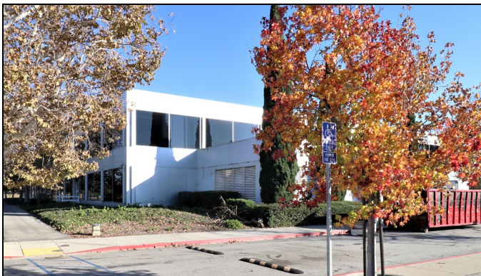
Northwest corner of the building showing addition, view southeast (11/18/22).
