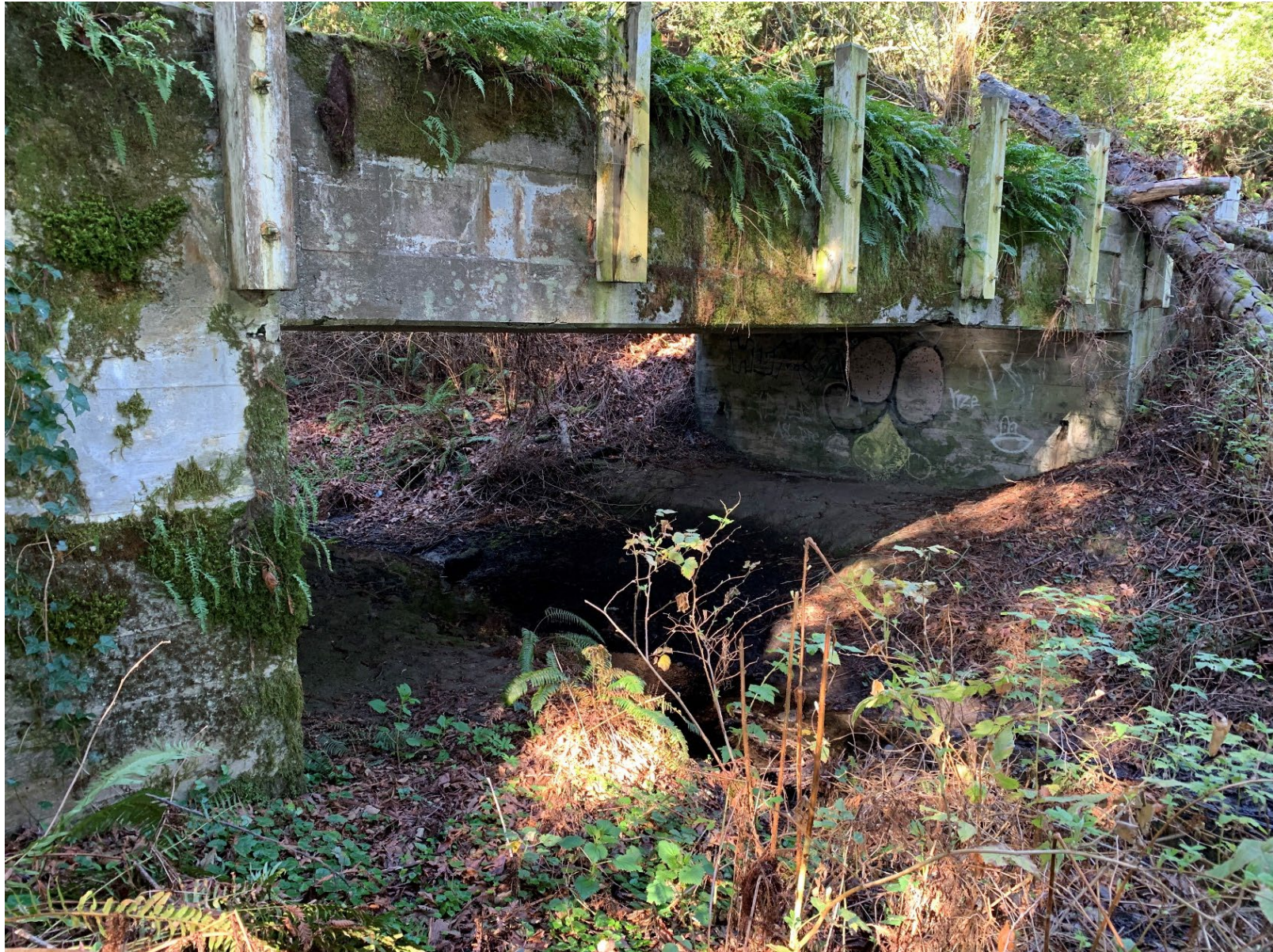
Figure 1. Old Bridge within Ward Creek approximately 100' downstream of project site.
