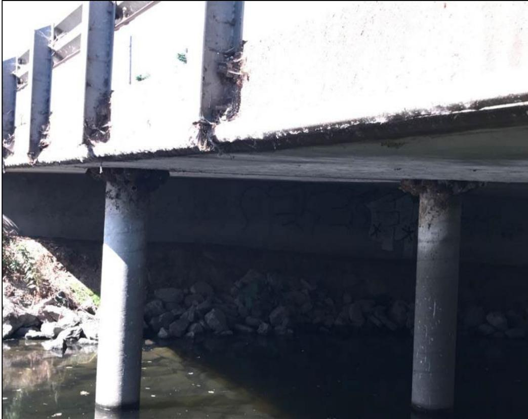
Looking south toward the south bank and bridge abutment reinforced with non-engineered rock slope protection (AECOM 2021b).
