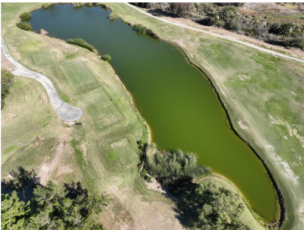
Photo of GCP-1 from air with service road and freshwater marsh in upper right.
