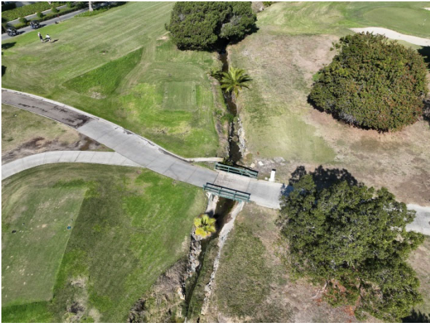
Photo of Drainage A channel from air south of Alga Road.
