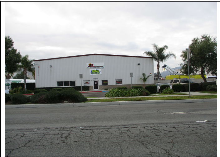
21. View of FR facility north of the Site.
