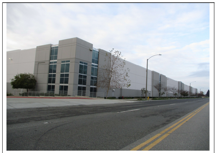
24. View of a warehouse building north of the Site.
