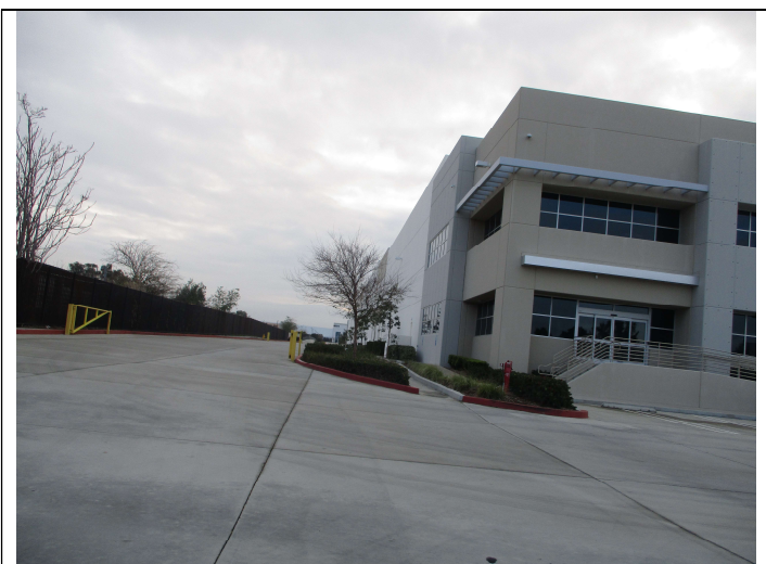
23. View of a warehouse building south of the Site.
