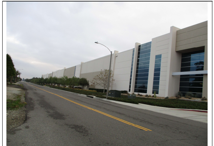
22. View of a warehouse building east across Catawba Ave.
