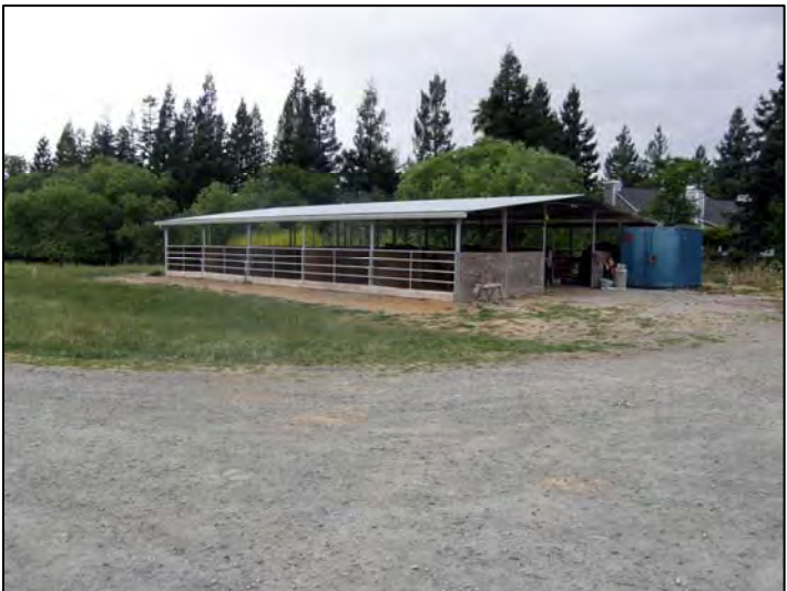
Looking west at northwest at horse stable
