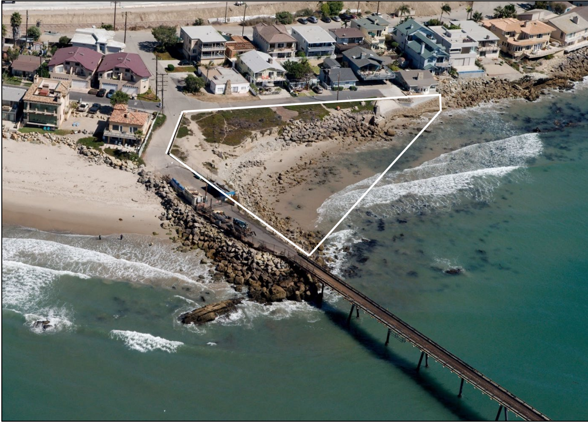
Figure 2. Aerial photograph of the abutment, causeway and the State Coastal Conservancy parcel. Approximate boundaries outlined in white (2013 photo from California Coastal Records Project – Kenneth and Gabrielle Adelman).
