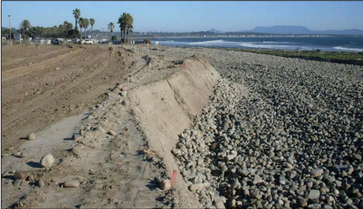
Figure 24 .Cobble berm under construction at Surfer’s Point.
