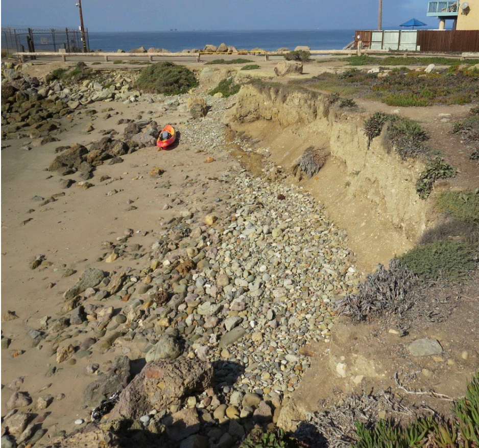
Figure 18. View of the flat upper portion of the SCC parcel and the bluff fronted by a cobble berm (October 2, 2022).
