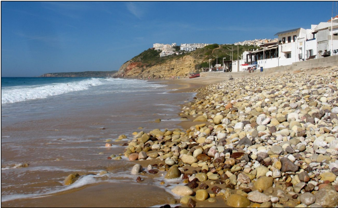
Figure 19. Natural cobble berm on the Algarve, Portugal.
