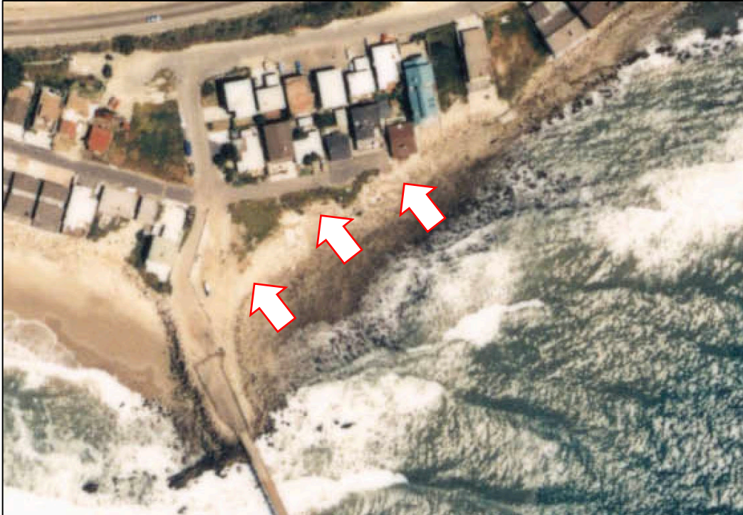
Figure 11. 1993 photograph. Recent wave action appears to have overtopped and moved the riprap seaward and eroded the coastal bluff landward at arrows.
