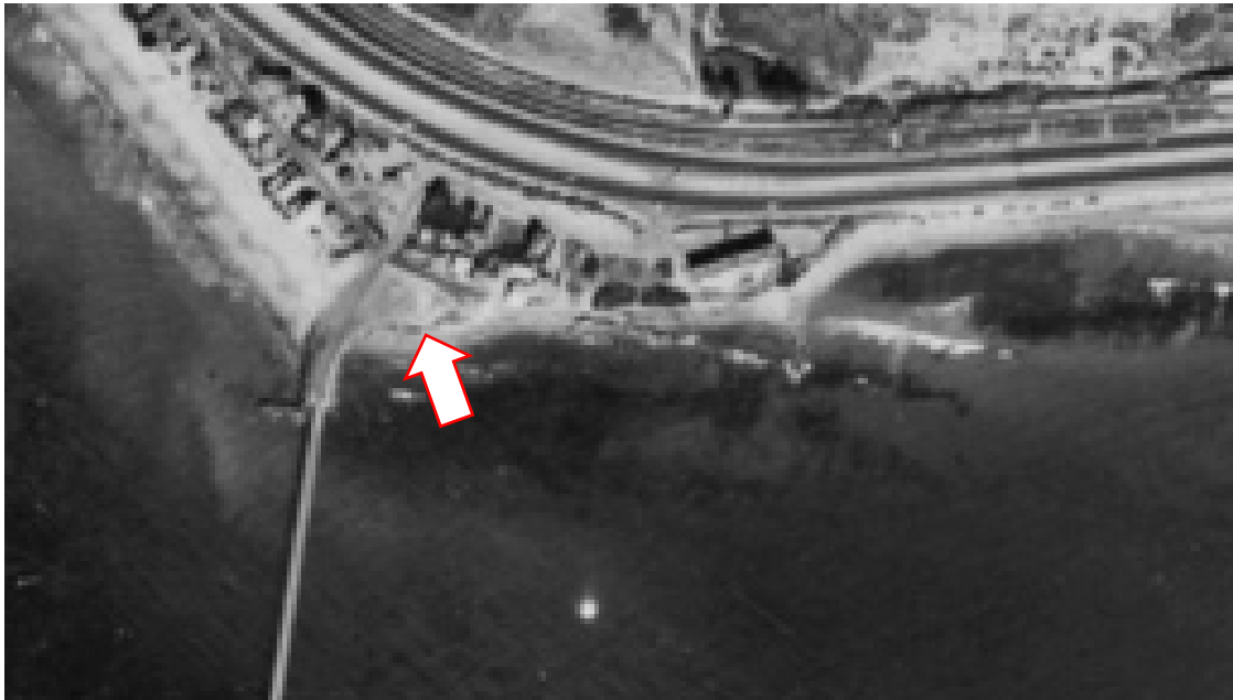
Figure 7. State Coastal Conservancy parcel in 1963 following 1959 construction of abutment and causeway. Dark area along the shoreline (arrow) appears to be rip rap that was placed in an arc extending from the abutment downcoast along the back beach.
