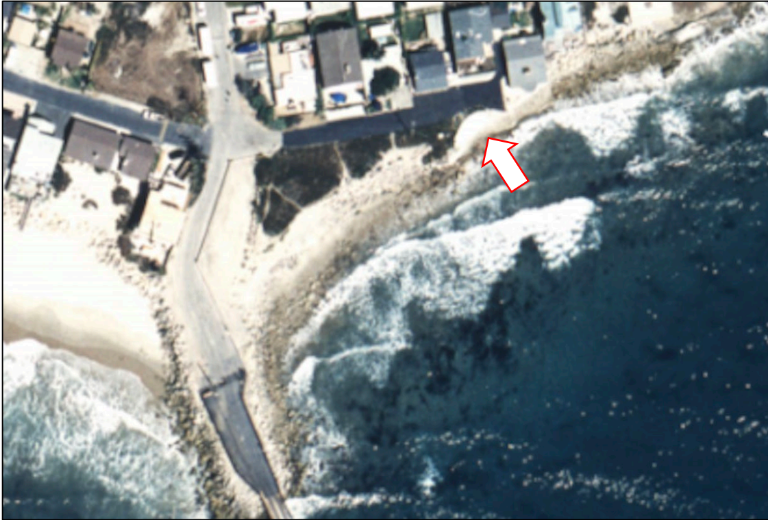
Figure 12. 2001 photograph showing eroded shoreline and curved-face concrete seawall at eastern edge of parcel (arrow).
