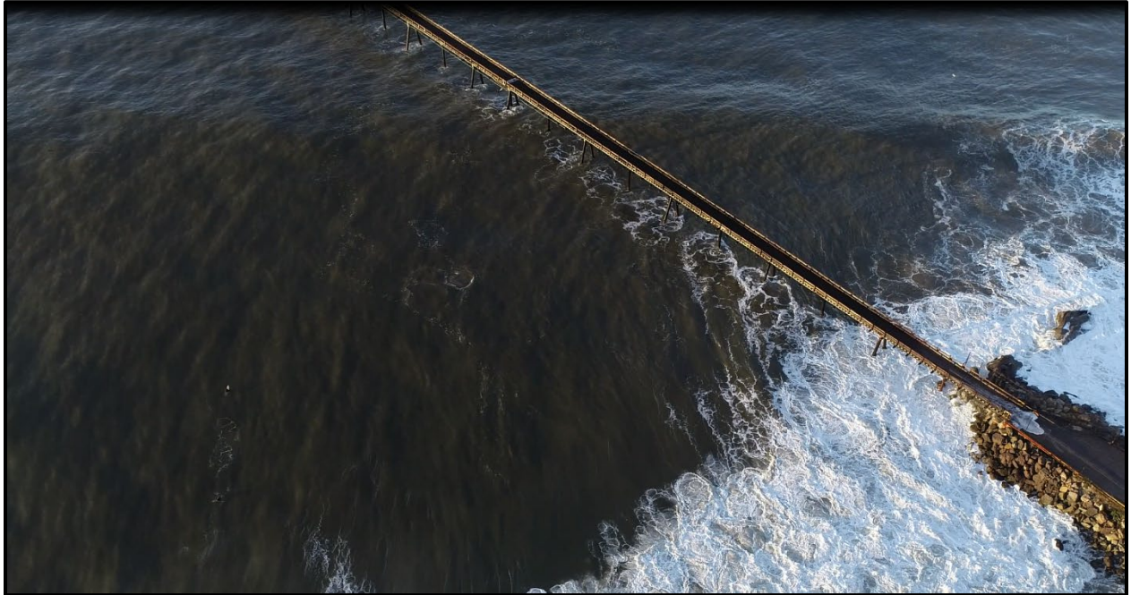
Figure 3-14. Frame from UAV Video Showing Waves Passing through Pier
