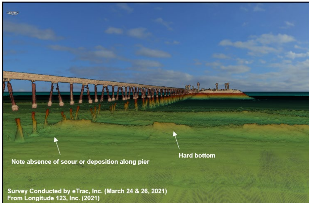
Figure 4-4. Sea Bottom at Rincon Pier
