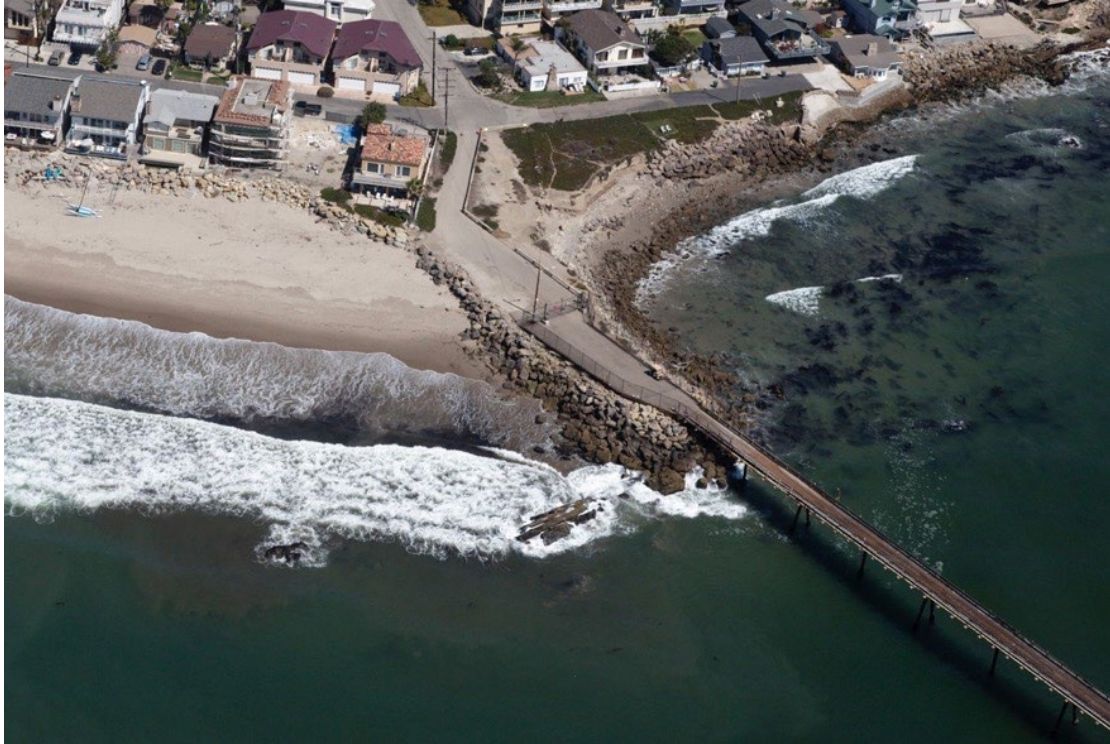
Figure 28. Close-up of the shoreward end of the causeway showing concave shape (2010 – California Coastal Records Project – Kenneth and Gabrielle Adelman).
