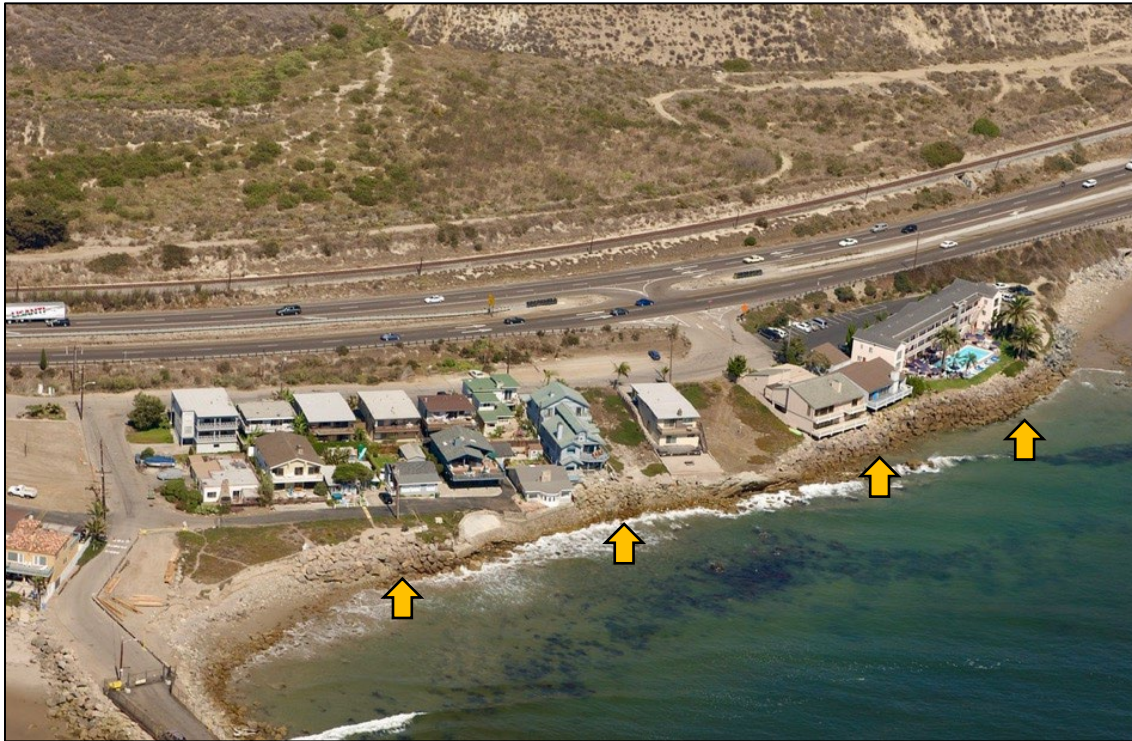
Figure 23. 2002 photo showing where riprap has been placed downcoast from the abutment.
