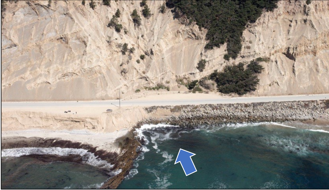
Figure 36b. Natural bedrock groin that has trapped sand upcoast (to the left) but produced erosion downcoast requiring the installation of riprap to protect State Highway 1 in northern Santa Cruz County (both photos: California Coastal Records Project- Kenneth and Gabrielle Adelman).
