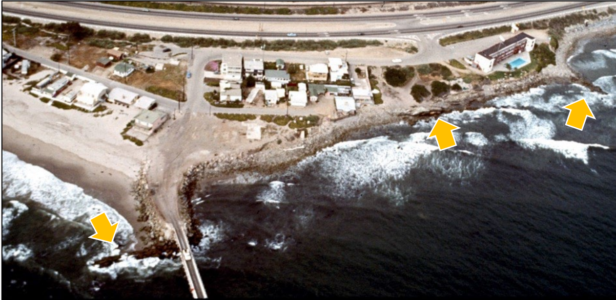
Figure 35. Concrete abutment and riprap was built seaward only as far as the bedrock outcrop in 1959 (arrow). There are additional rock outcrops downcoast (arrows) (Photo 1972 California Coastal Records Project – Kenneth and Gabrielle Adelman).
