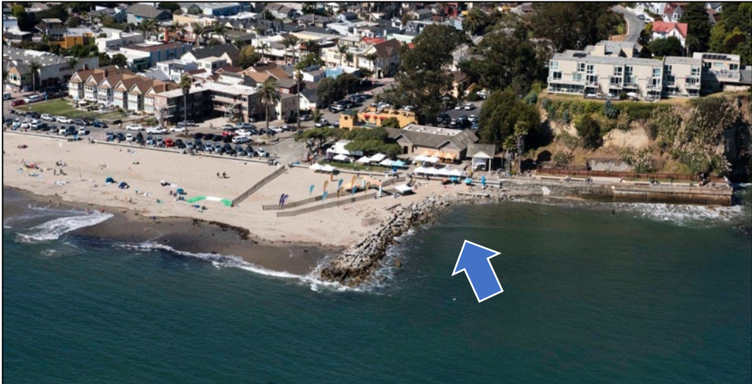
Figure 36a. The Groin Effect. Groin constructed in city of Capitola in northern Monterey Bay which has retained beach to the left but erosion is occurring downcoast to the right.
