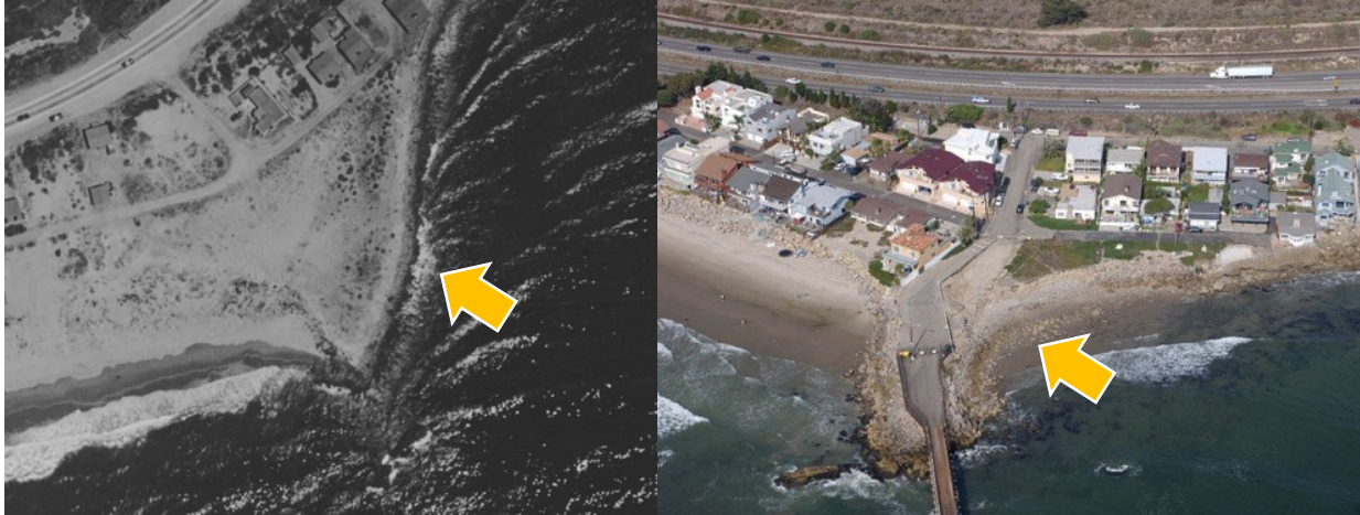
Figure 24. Comparison of 1927 image and 2004 image showing difference in shoreline area immediately downcoast of the abutment.
