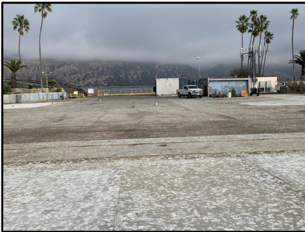
Island Interior Looking North Towards Causeway Entrance
