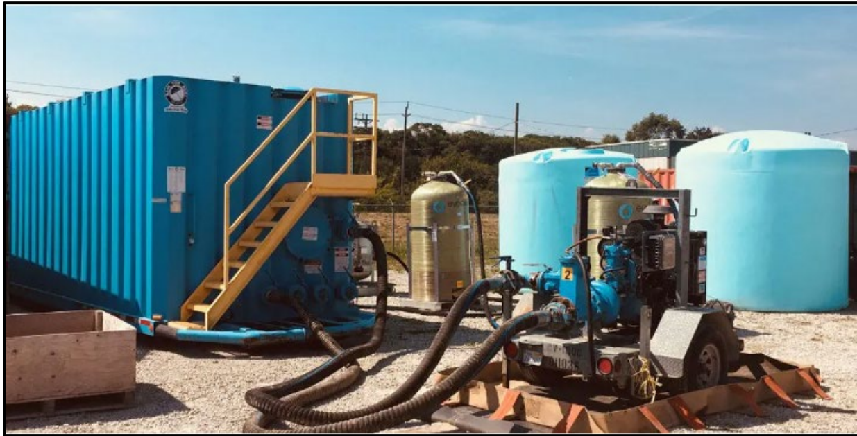
Figure 2-26. Example Groundwater Pump and Treat System
