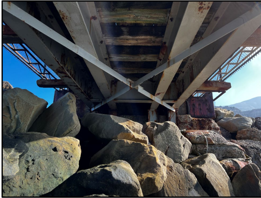
Figure 2-6. Rincon Island Causeway Abutment
