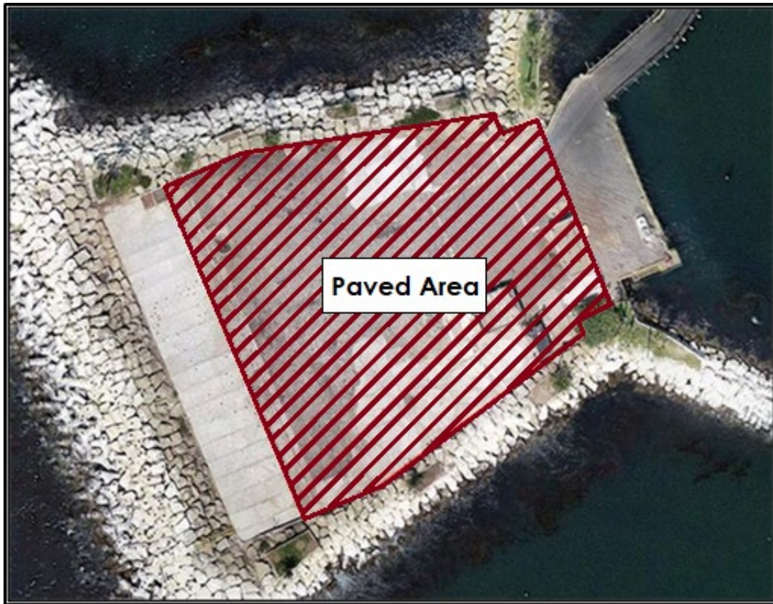
Figure 2-17. Rincon Island Asphalt Pavement
