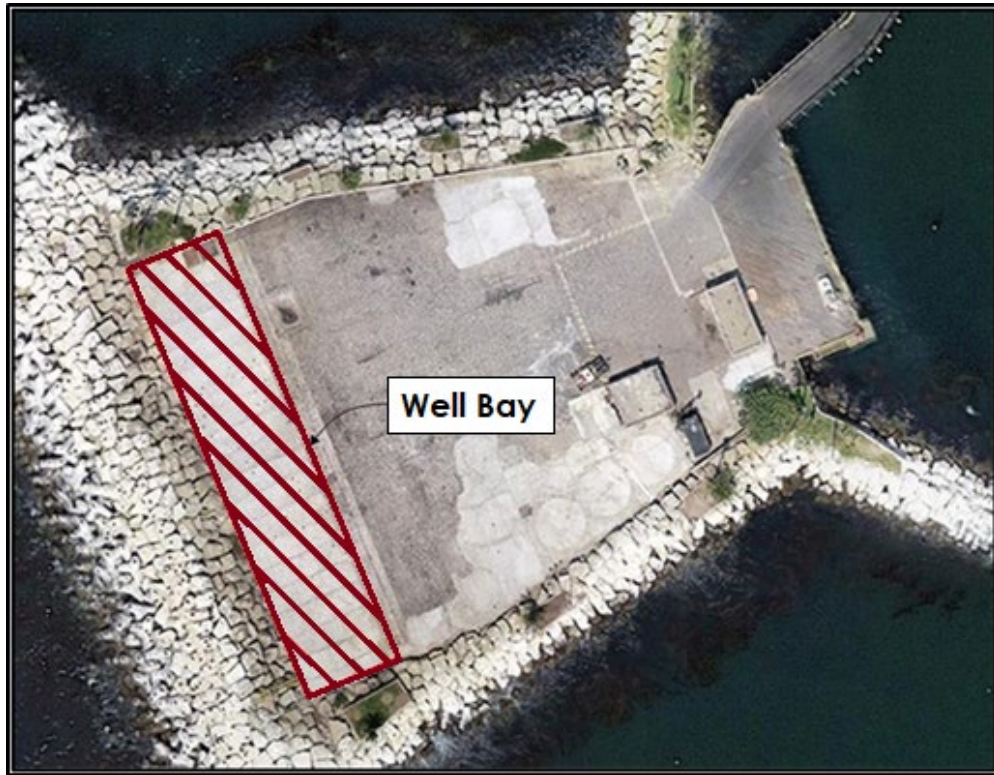
Figure 2-15. Rincon Island Well Bay Concrete Deck
