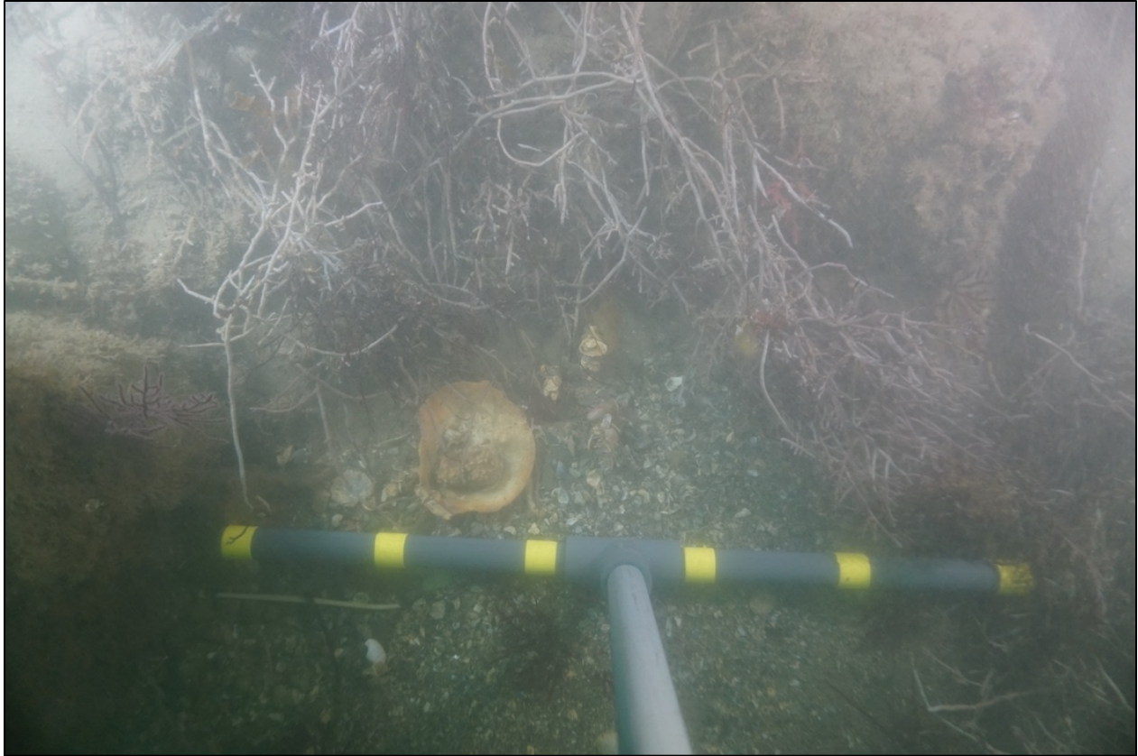
Figure 22. Scallop Shell at the Base of the Armor Revetment
