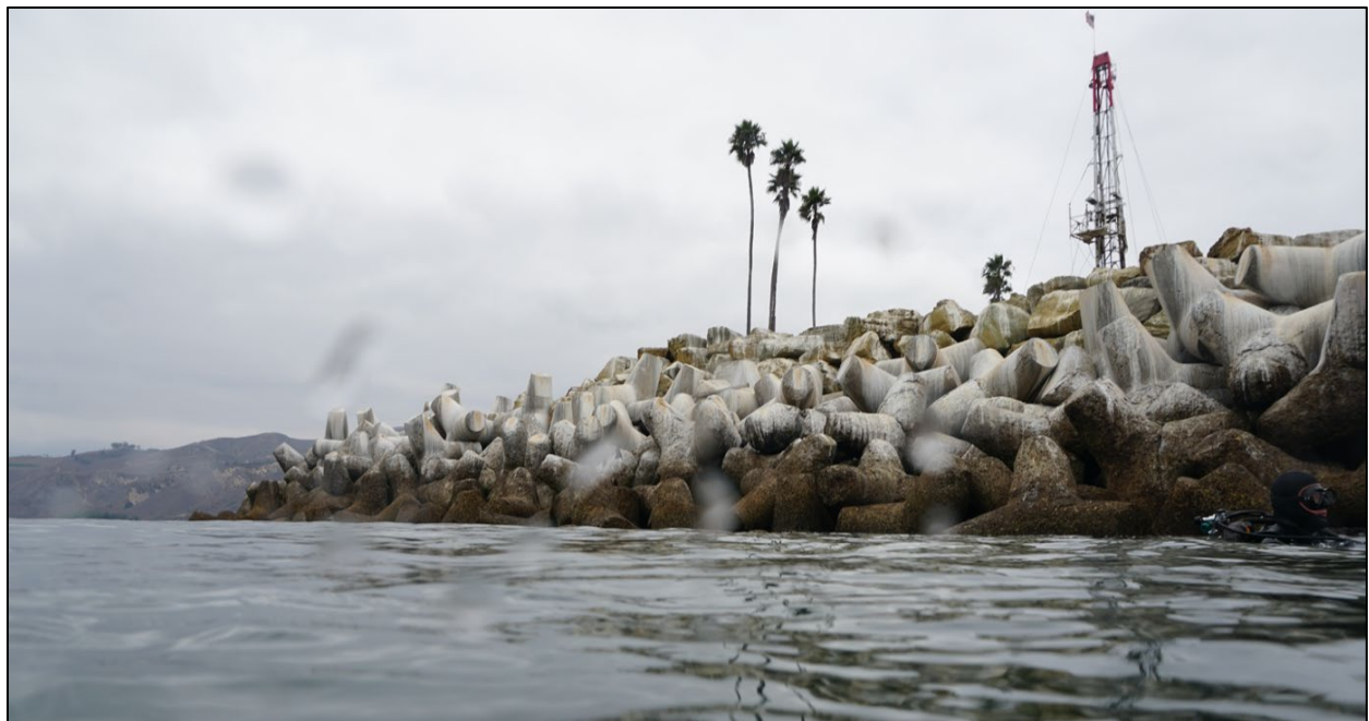
Figure 3. West Side Tetrapods from the Sea Surface
