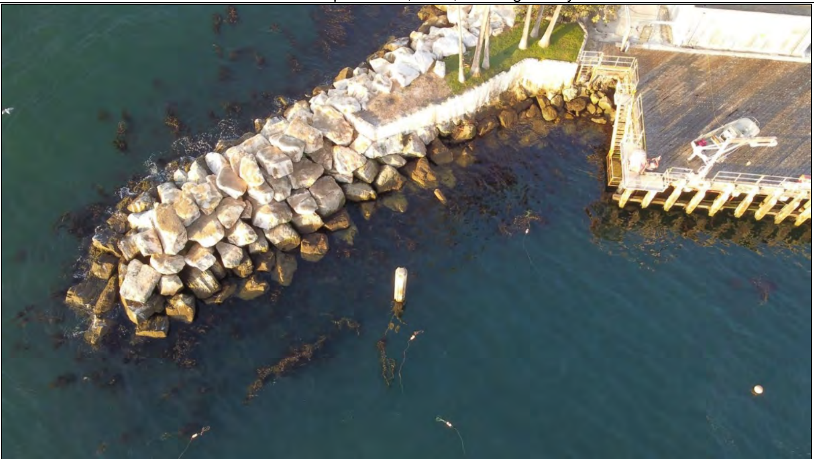
Photo 3b: October 28, 2022, morning survey.
