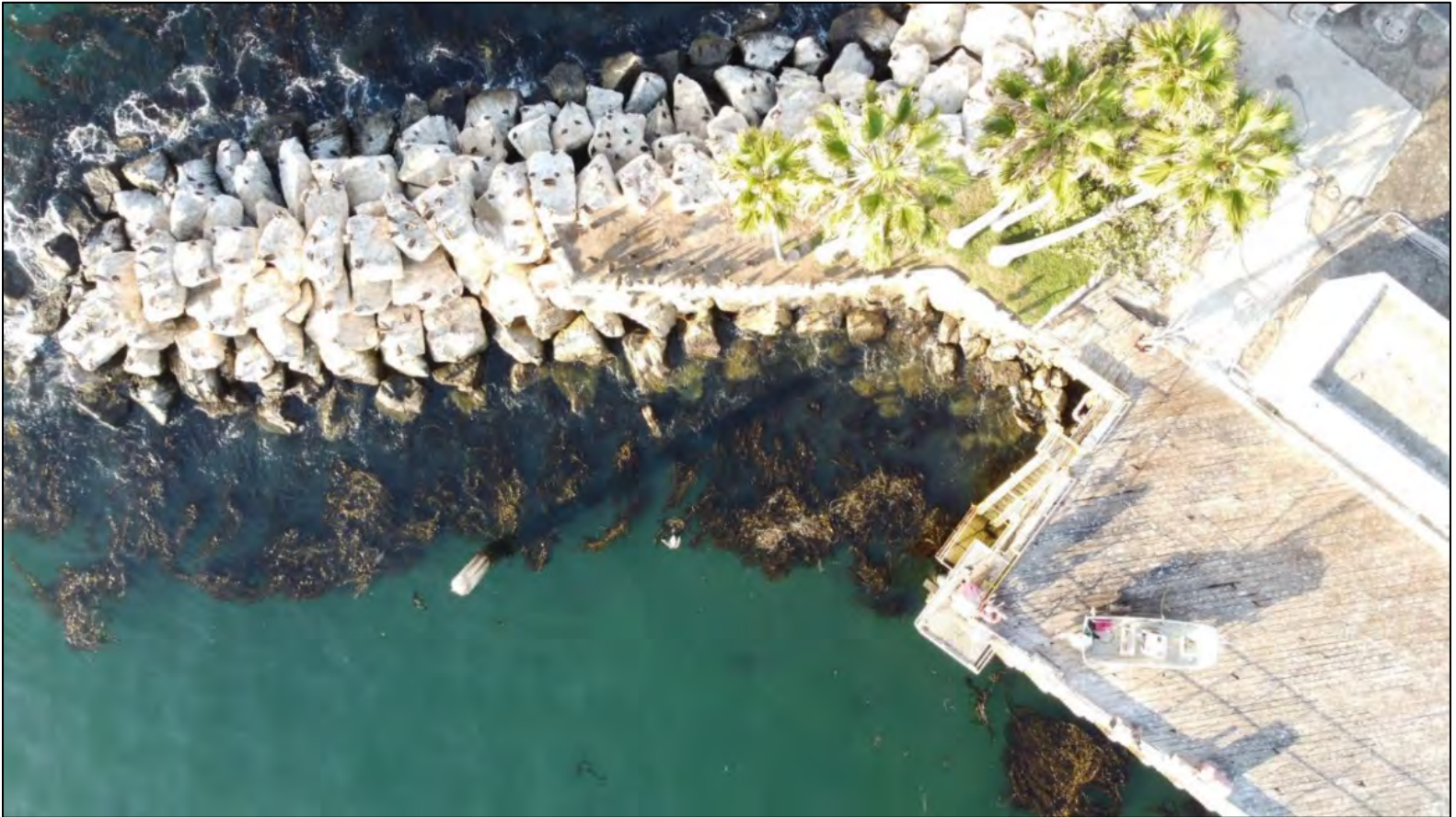
Photo 3a: September 6, 2022, morning survey.
