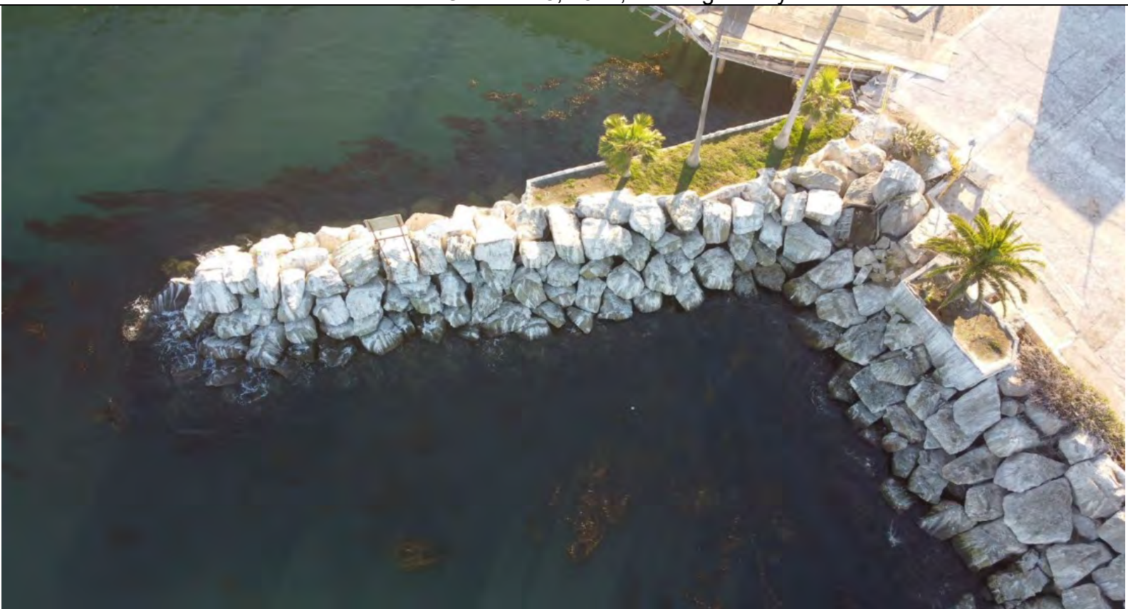
Photo 7c: December 21, 2022, morning survey.
