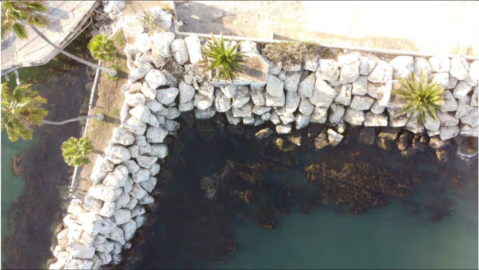
Photo 7a: September 6, 2022, morning survey.
