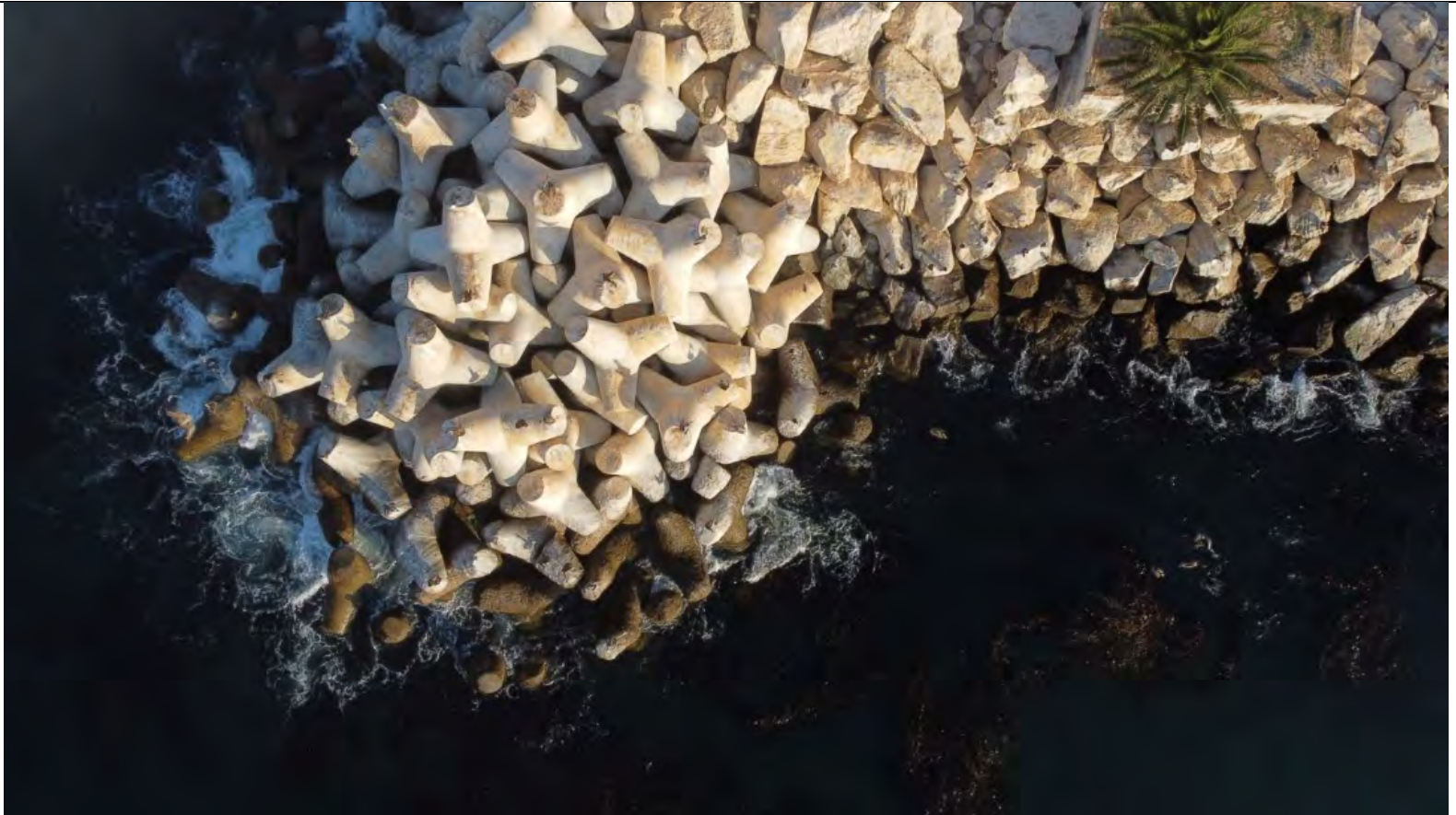
Photo 9a: September 6, 2022, morning survey.
