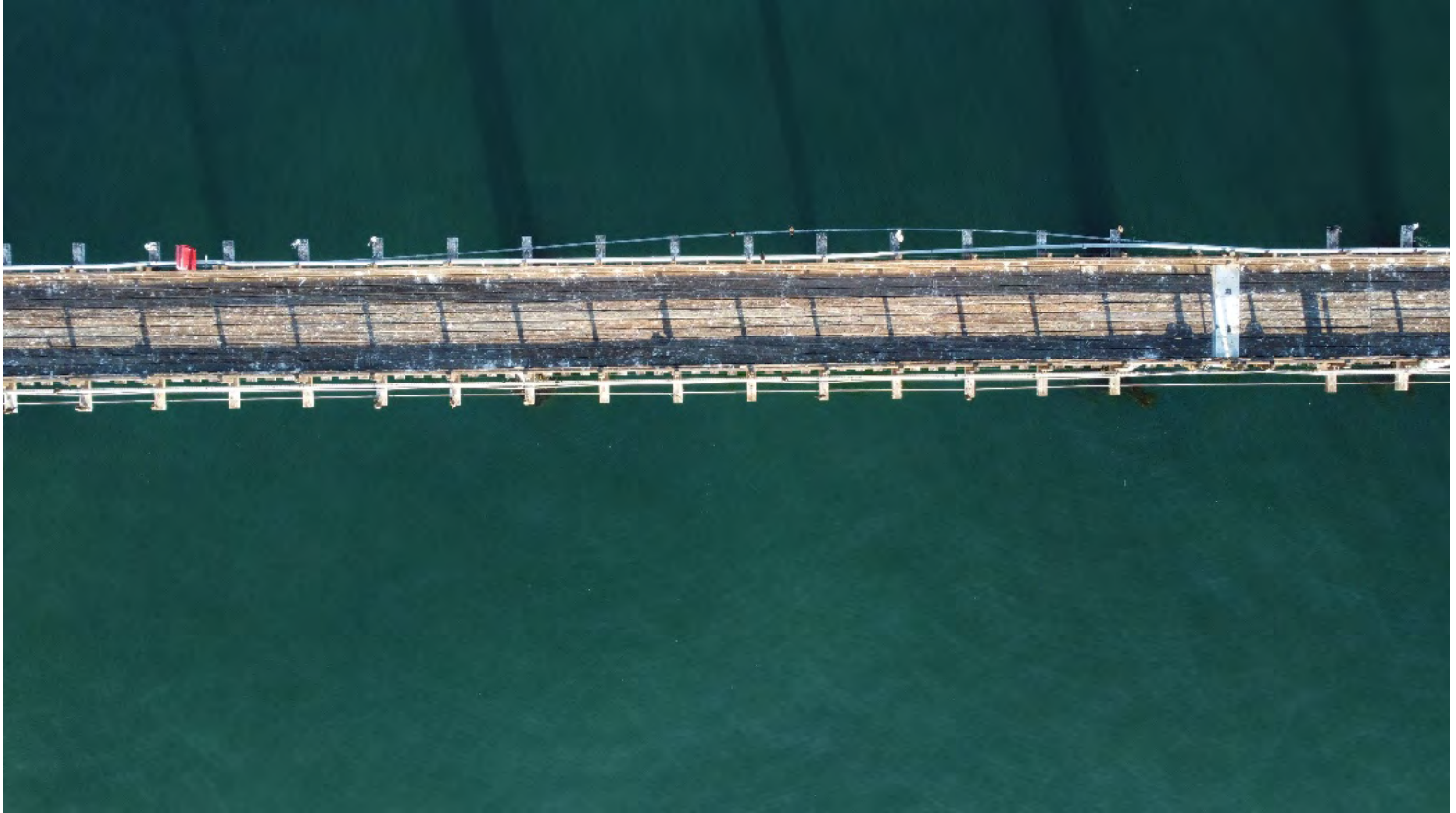
Photo 1a: September 6, 2022, morning survey.
