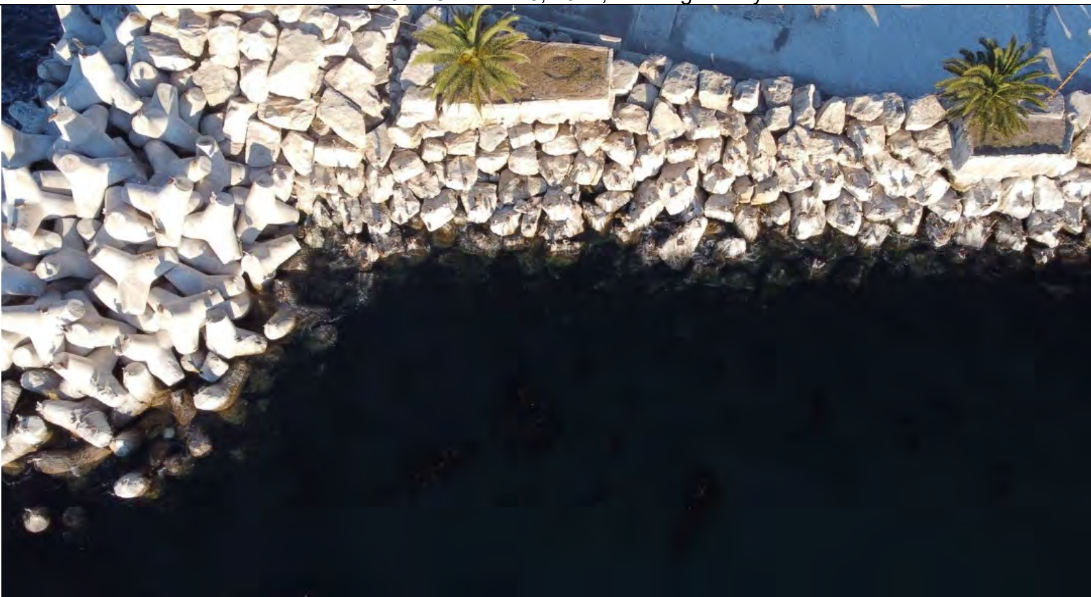
Photo 9c: December 21, 2022, morning survey.
