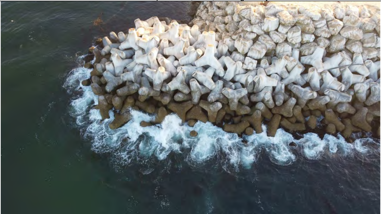
Photo 5b: October 28, 2022, morning survey.
