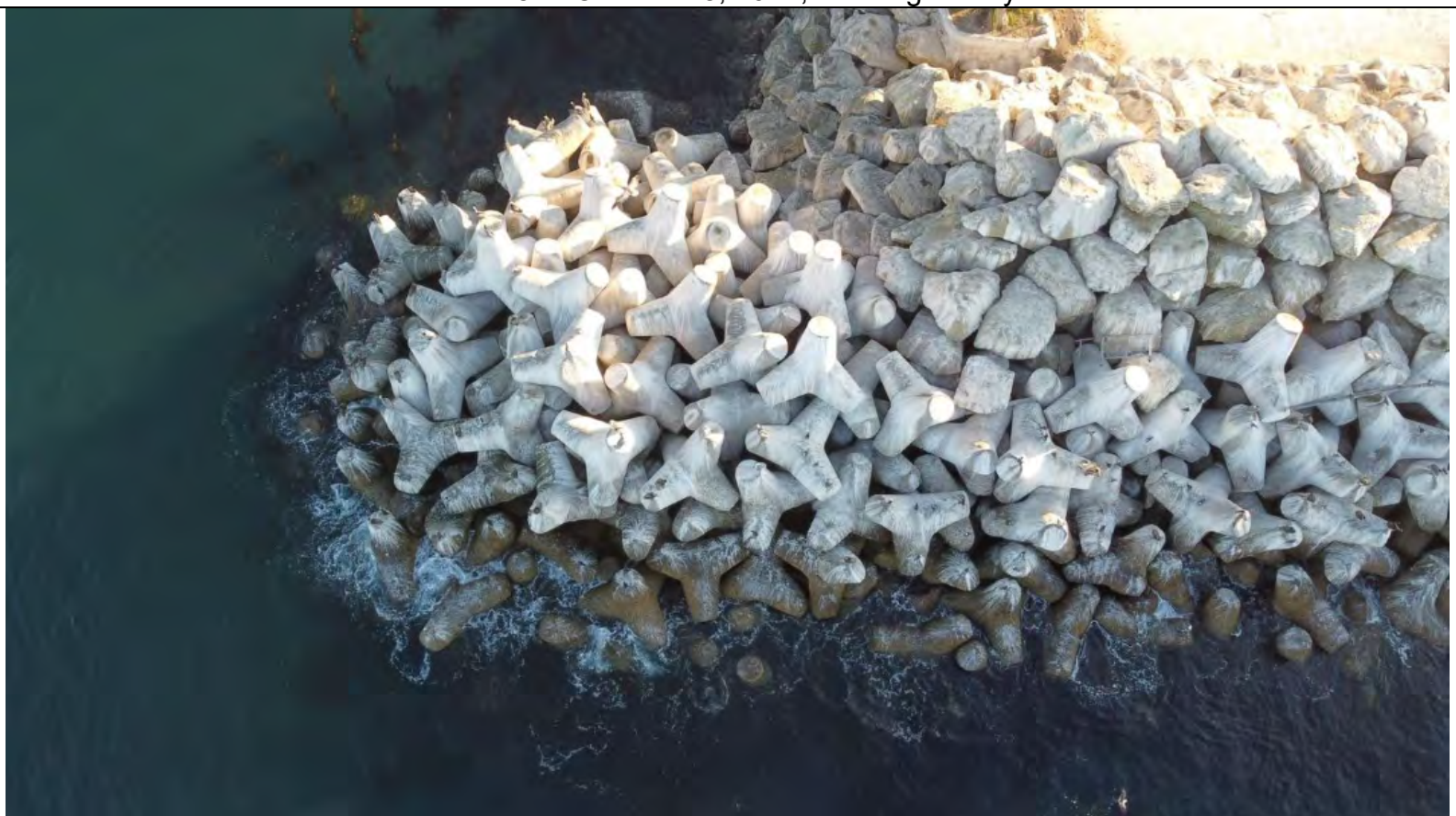
Photo 5c: December 21, 2022, morning survey.
