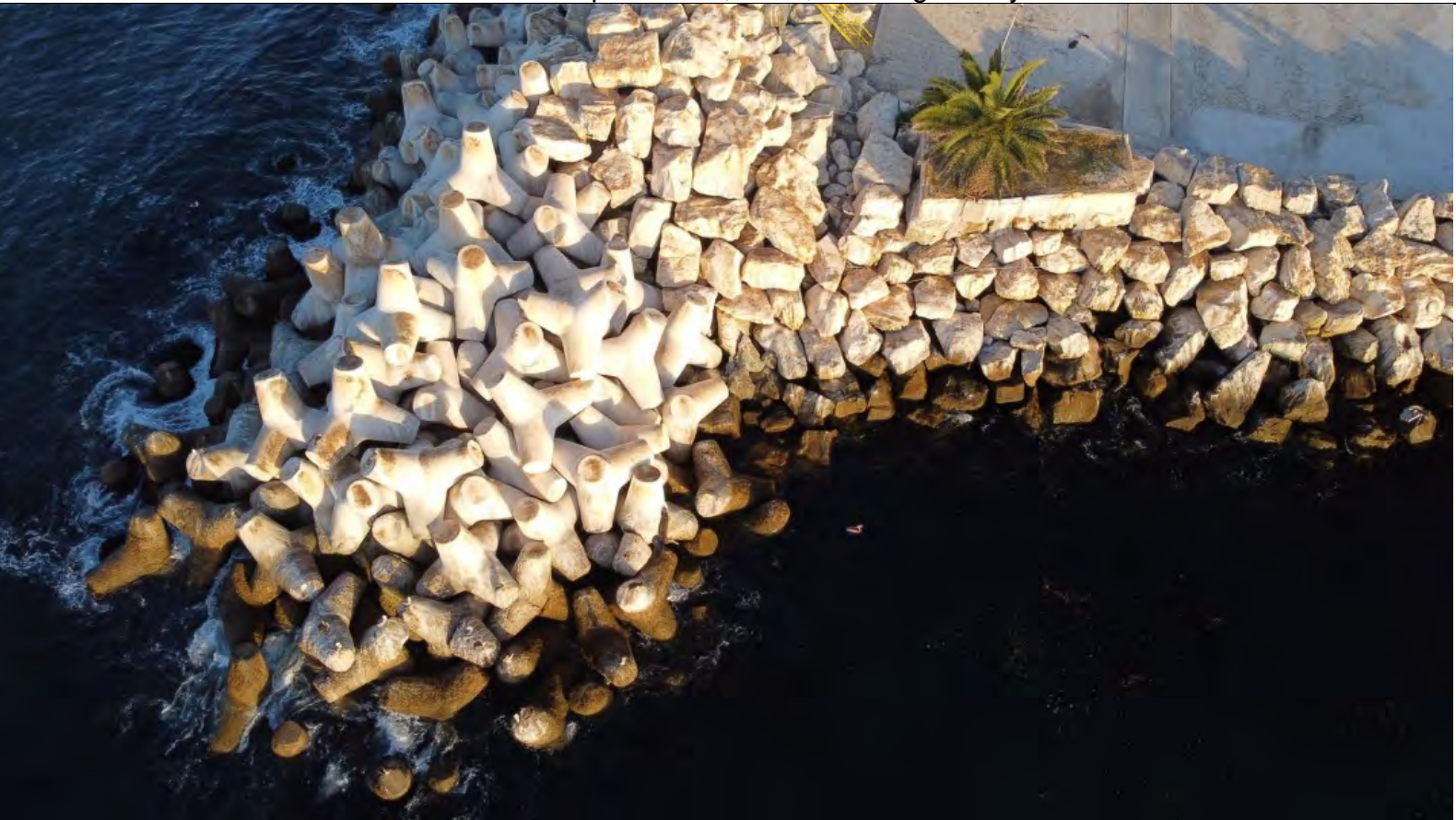
Photo 9b: October 28, 2022, morning survey.
