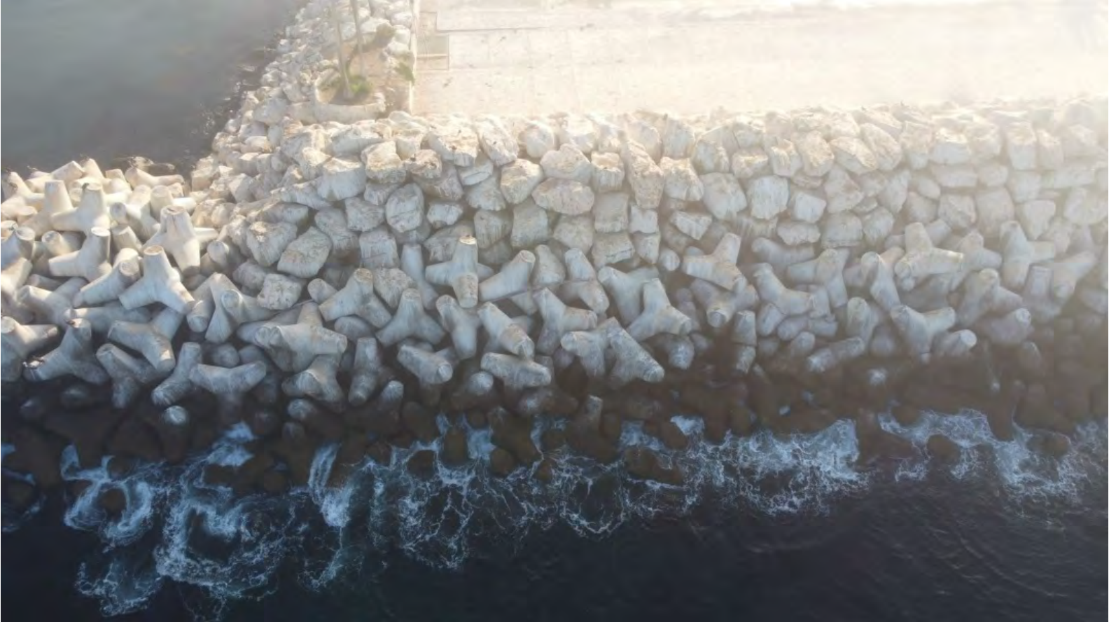
Photo 5a: September 6, 2022, morning survey.
