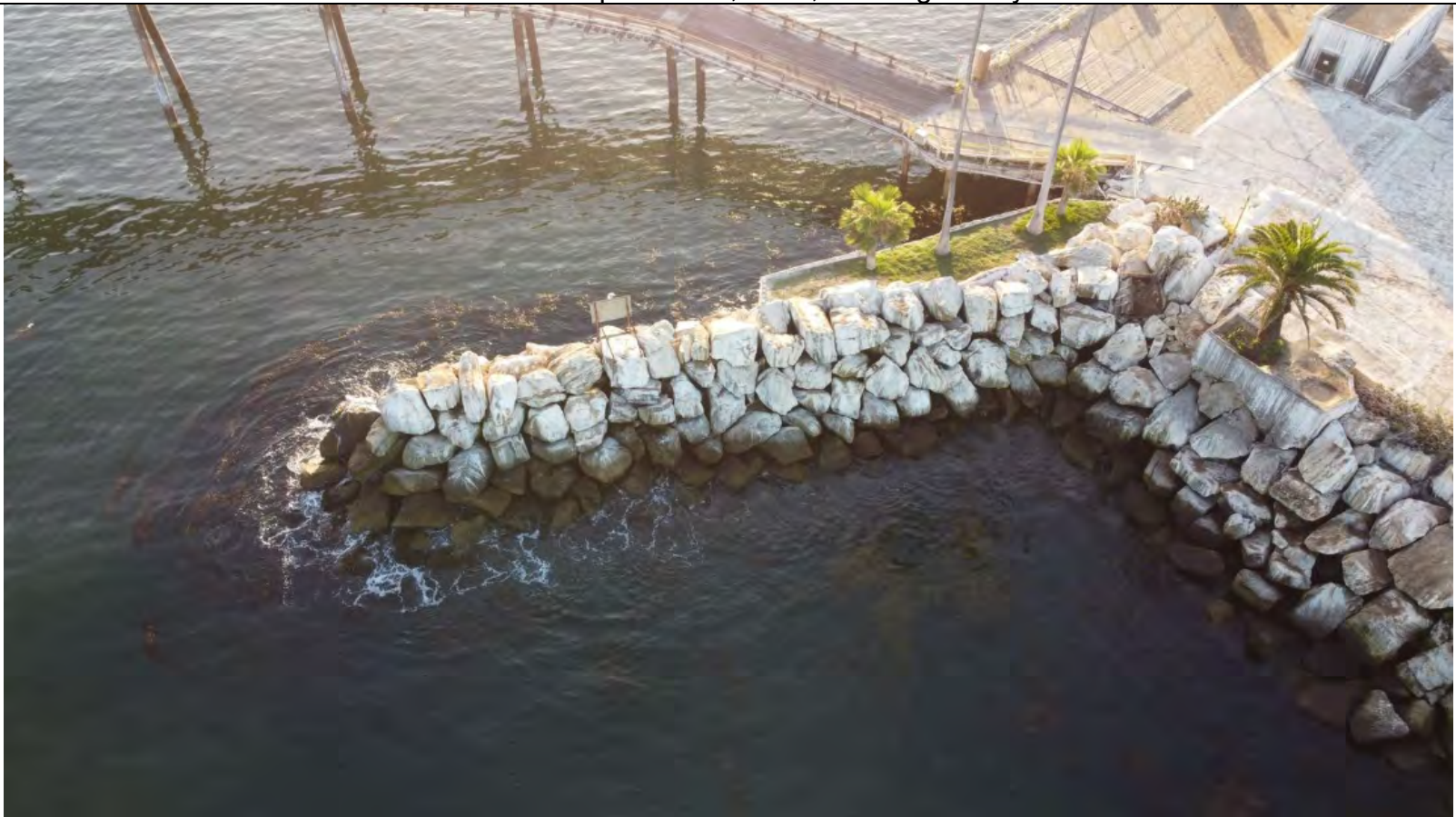
Photo 7b: October 28, 2022, morning survey.
