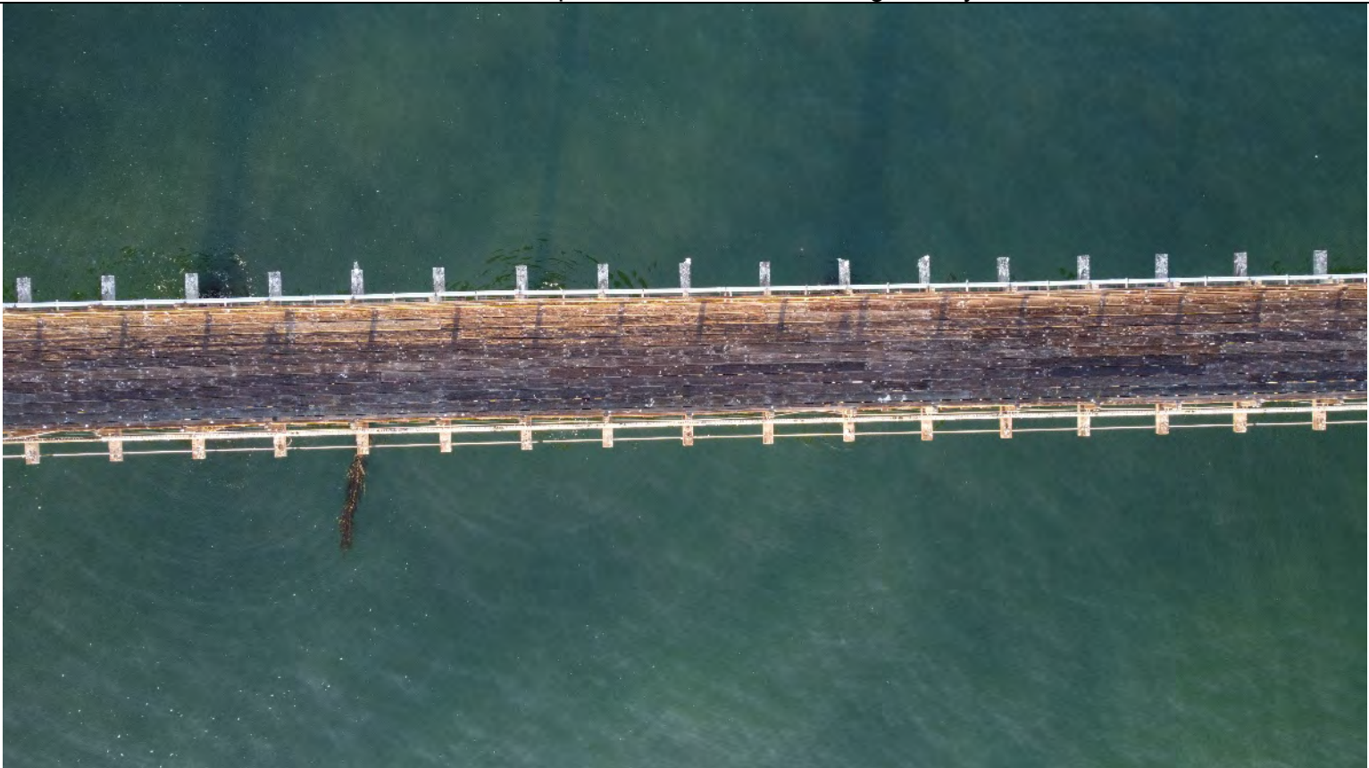
Photo 1b: October 28, 2022, morning survey.
