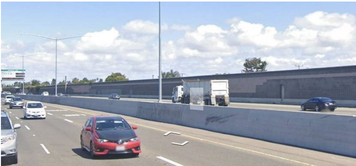
Figure 1-4. Example Concrete Barrier Type 60M with Optional Lighting Attached
