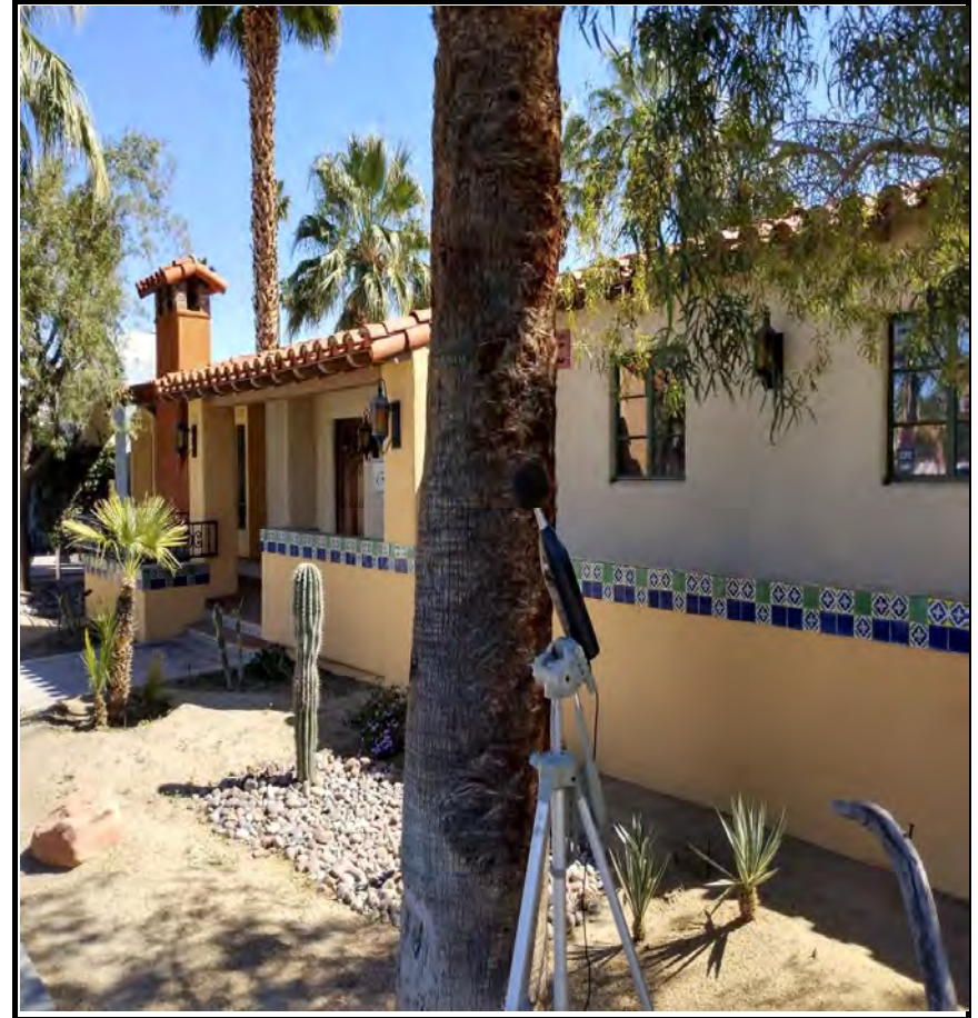
STNM3 looking SE towards building 515 N Palm Canyon Drive C, Palm Springs.
