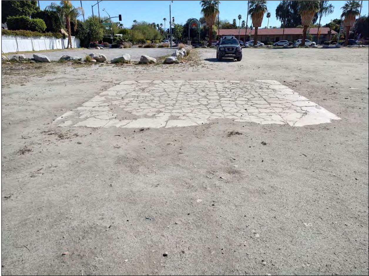
Figure 11. Concrete pad in the project area. (Photograph taken on March 8, 2022; view to the east)
