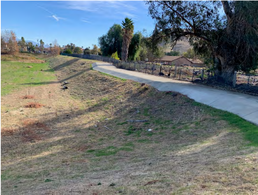
Photograph 3: Looking east from southwest corner of the basin.
