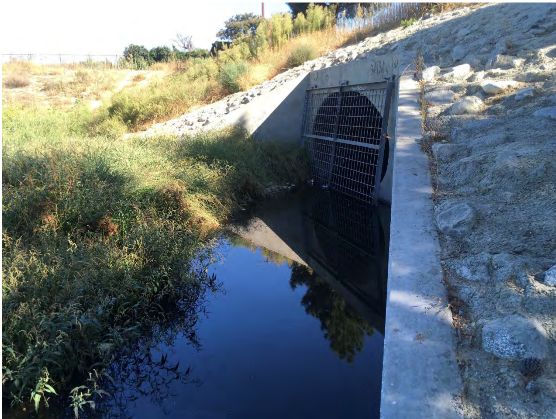
Photo 6. Large inlet grate east
