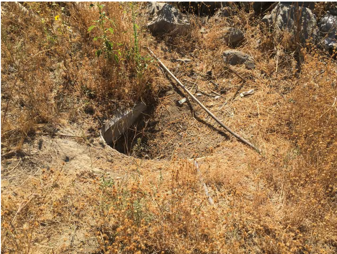
Photo 8. Small inlet drain north
