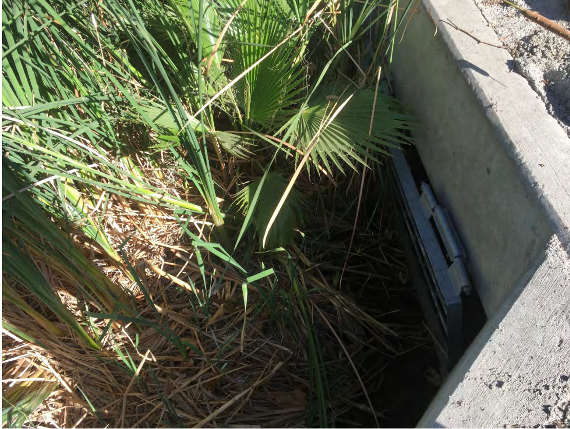
Photo 5. Small inlet grate east
