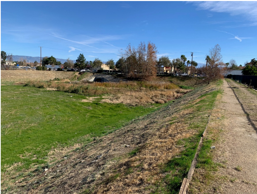
Photograph 2: Storm drain discharge point and aquatic vegetation on the eastern boundary of the site.
