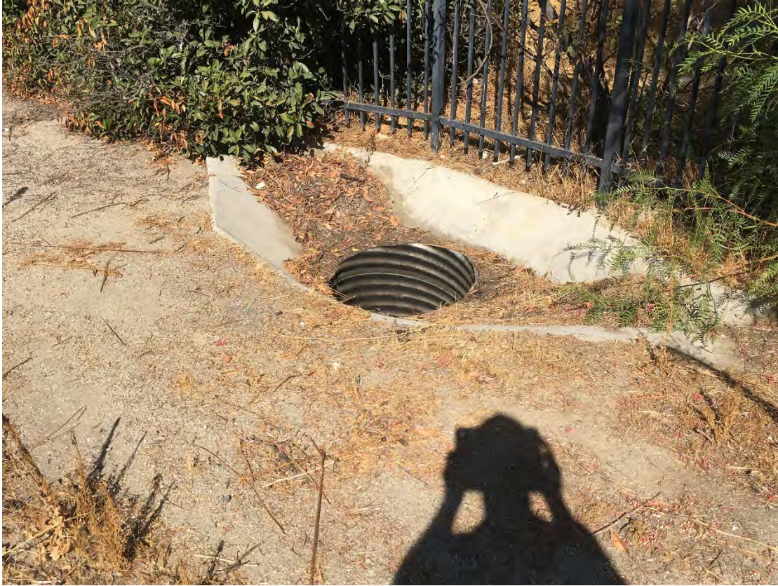
Photo 7. Small inlet drain north
