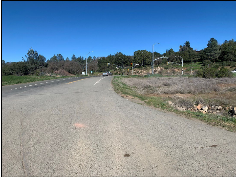
Existing SR 53/18 th Avenue Intersection
