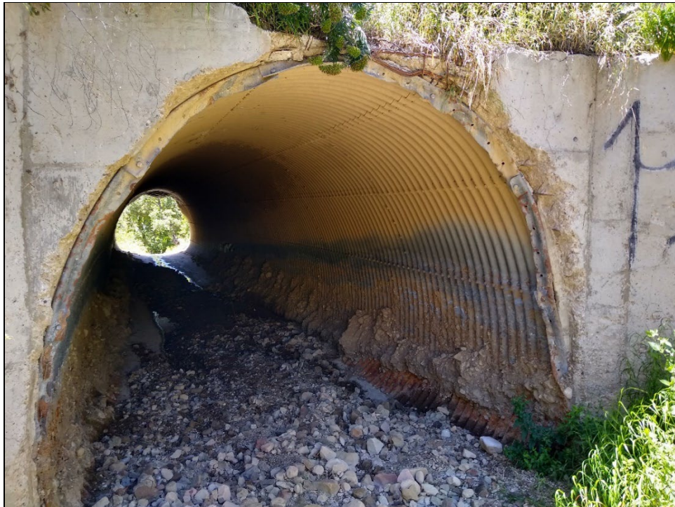
Photo 8. View of culvert beneath Park Lane facing south.
