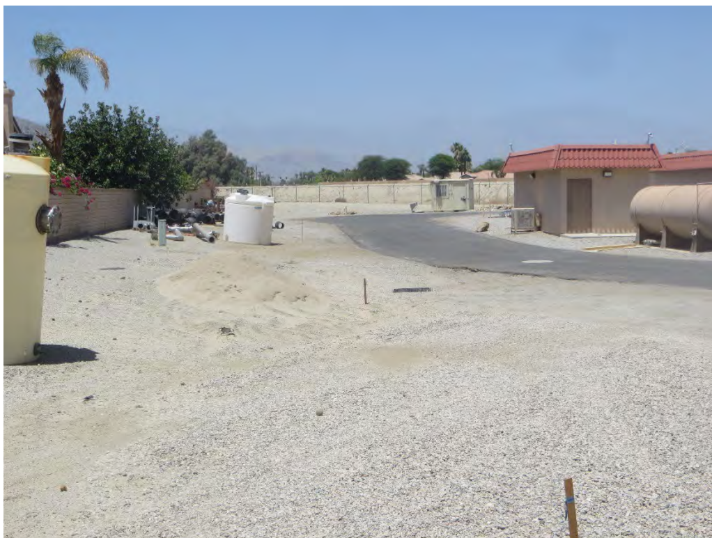
Photograph 6: From the eastern limits of the project site looking west along the existing Valley Sanitary District facility.
