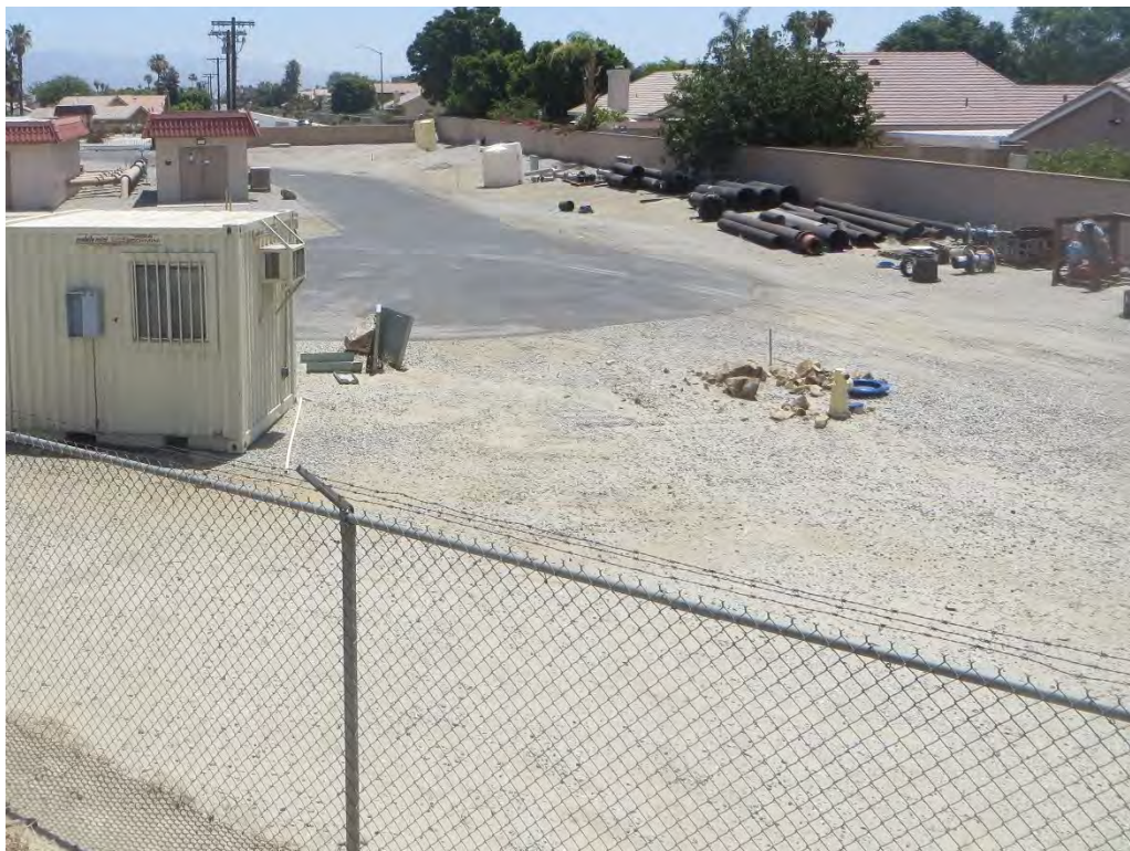
Photograph 5: From the eastern edge of the Coachella Valley Stormwater Channel looking west across the existing Valley Sanitary District facility.
