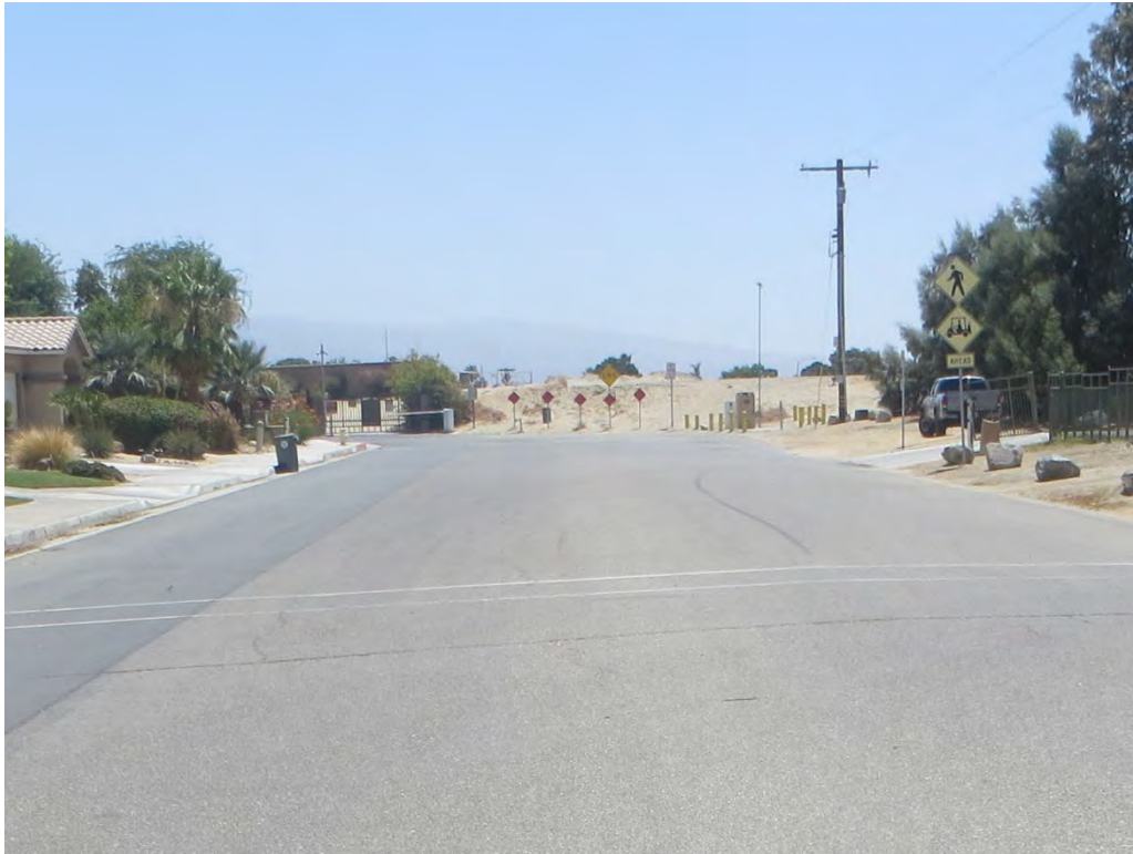
Photograph 1: From the western limits of the project site looking east along Westward Ho Drive.
