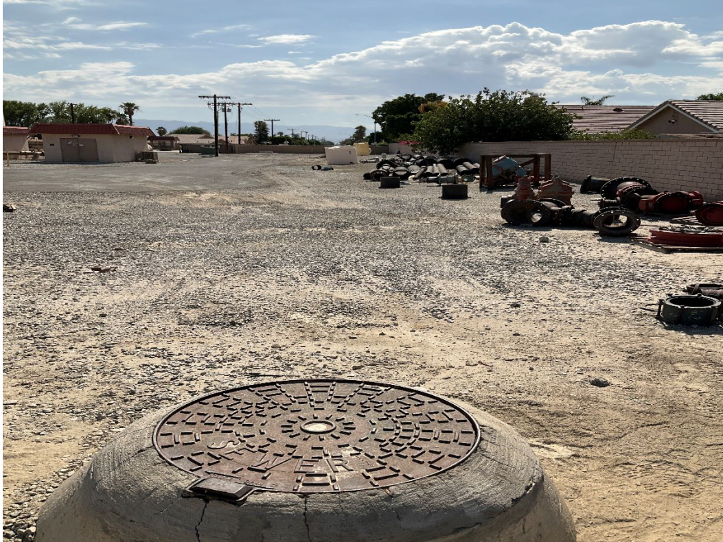
Figure 5-2. Overview of manhole in eastern Project area where tie-in will occur, facing east.
