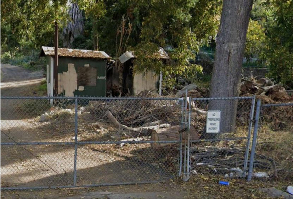
Figure 1. Old sheds in Project Planning Area 2.
