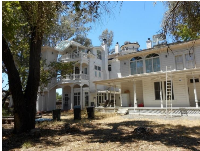
Photograph No. 8: North Elevation of Turtletaub Addition.
