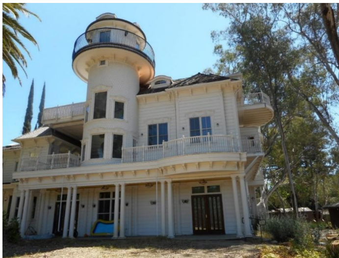
Photograph No. 5: West Elevation of Turtletaub Addition.
