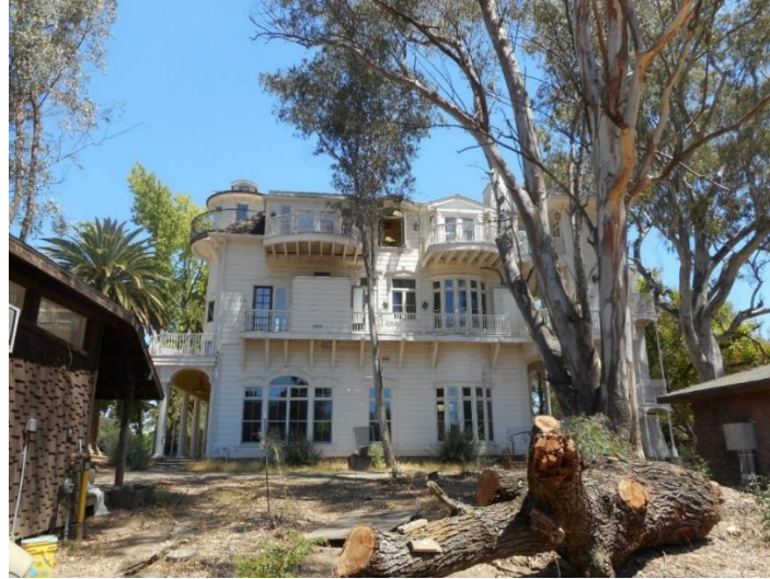
Photograph No. 6: South Elevation of Turtleaub Addition.
