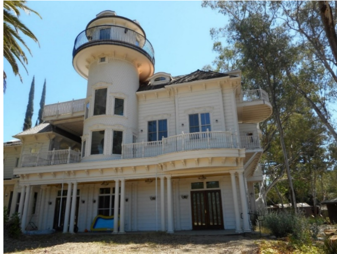
Photograph No. 5: West Elevation of Turtletaub Addition
