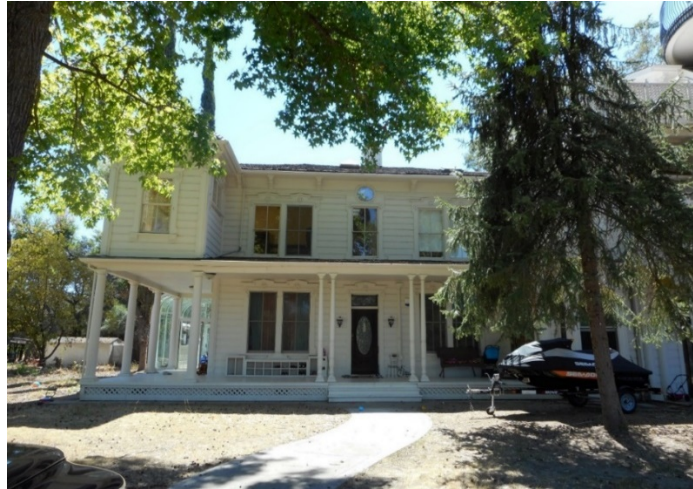
Photograph No. 1: West Elevation of c. 1875 Residence
