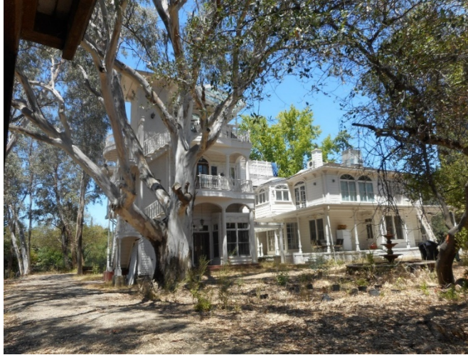
Photograph No. 7: East Elevation of Turtletaub Addition
