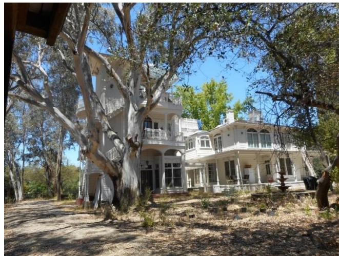
Photograph No. 7: East Elevation of Turtleaub Addition.
