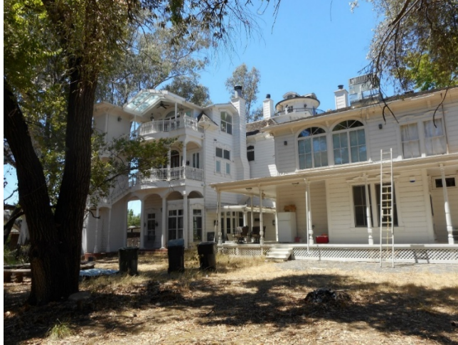
Photograph No. 8: North Elevation of Turtleaub Addition
