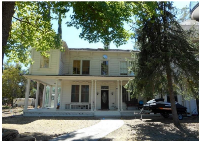
Photograph No. 1: West Elevation of c. 1875 Residence.
