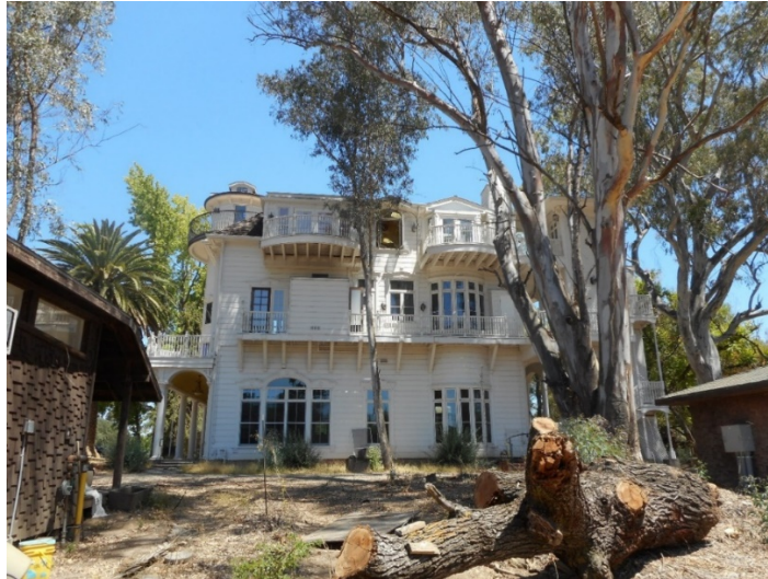
Photograph No. 6: South Elevation of Turtletaub Addition
