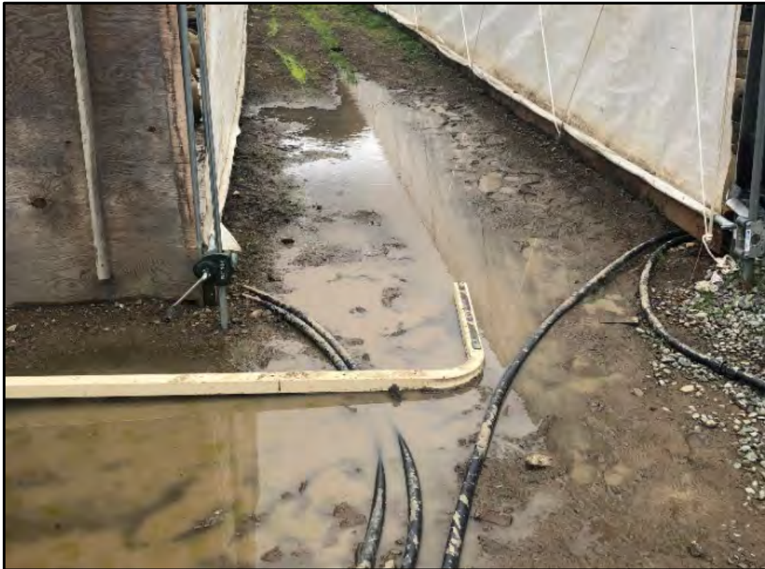
Figure 7- Standing Water was Observed in the Cultivation Area.
