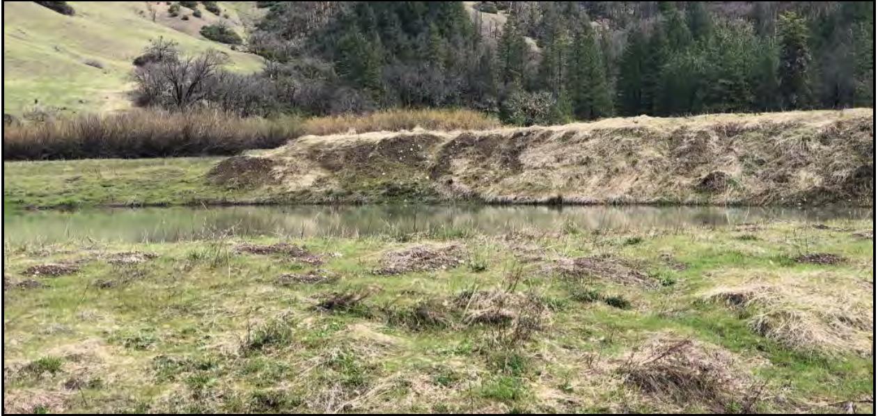
Figure 15- The Pond and Associated Embankment Identified on the Property.
