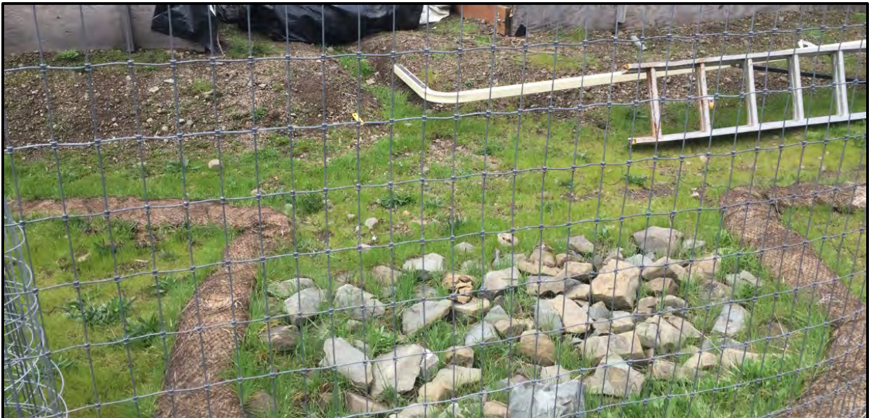
Figure 6- Wattles and Sediment Catchment Basins were Identified Downslope of the Cultivation Area.
