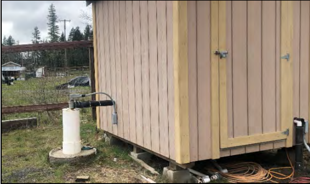
Figure 21- One of the Groundwater Wells Identified on the Property.
