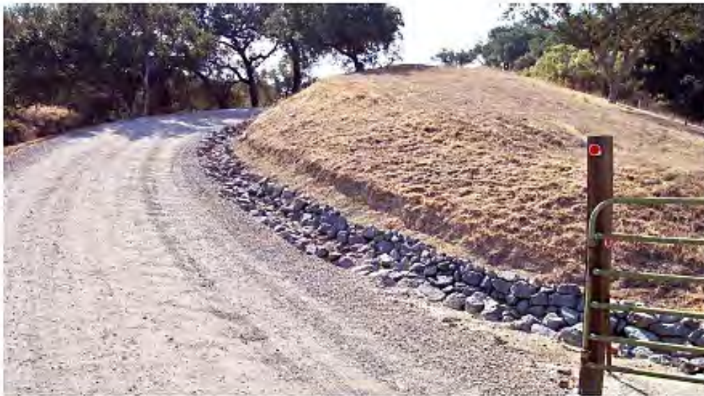
FIGURE 184. Rock armored ditches, if constructed with proper rock sizes, rock gradations and U-shaped channel form, can prevent ditch downcutting and erosion, but also inhibits easy ditch maintenance using machinery. Rather than armoring or installing check dams in ditches, it is usually best to reduce the volume of flow by installing additional ditch relief culverts.
