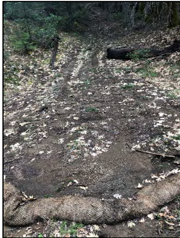
Figure 11- Portions of the Access Road were Steep and Exhibited Rutting. A Wattle was in Place to Disrupt and Prevent the Concentration of Sheet Flow.
