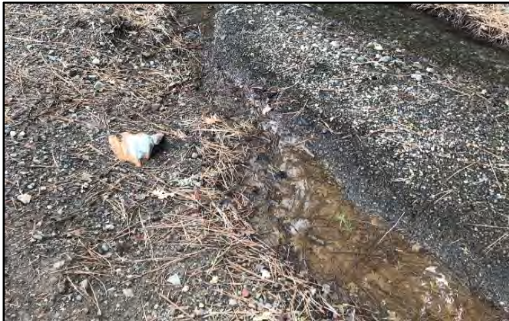
Figure 13- A Ditch Relief Culvert Identified on the Property.
