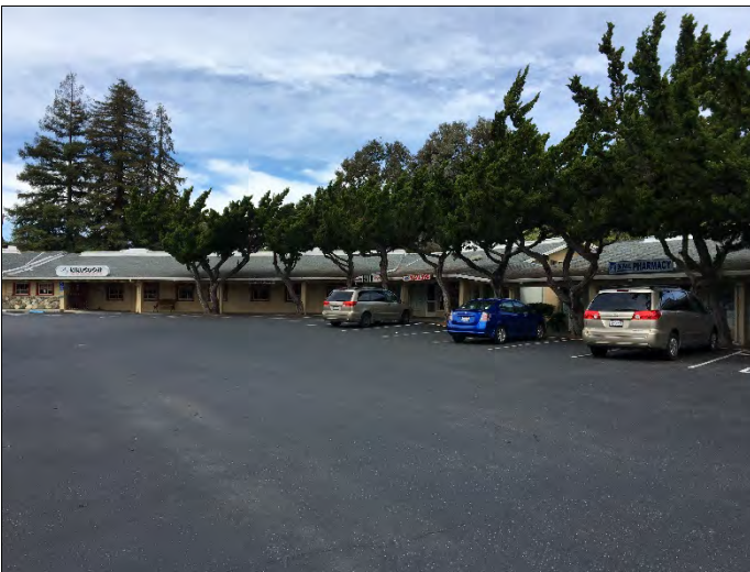
3. View of the south side of the subject property.
