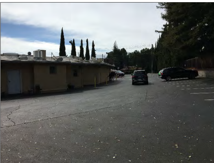
5. View of the west side of the subject property.
