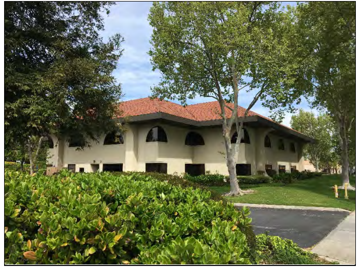
20. View of adjacent property to the north.
