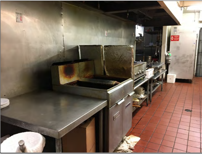
19. Interior view of the restaurant kitchen.
