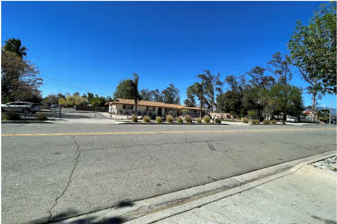
Photograph No. 1: Site, looking northwest.
