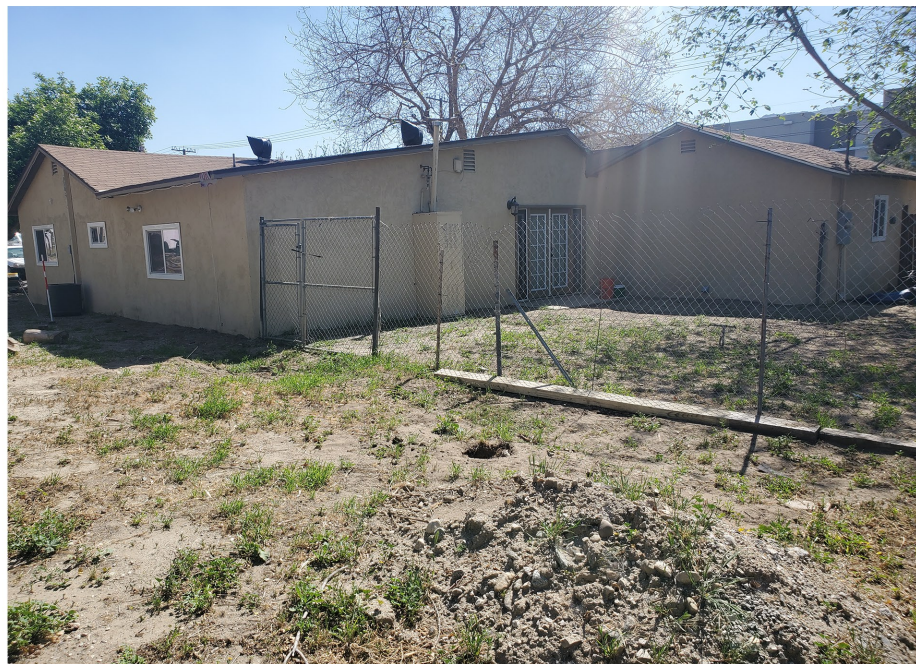
Plate 3.3–61: North (left) and west (right) façades of the 16228 Santa Ana Avenue building, facing southeast.
