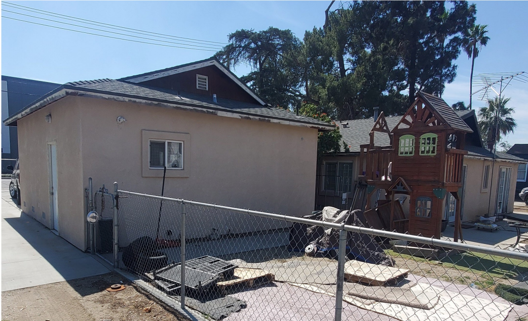
Plate 3.3-38: North façade of the 16156 Santa Ana Avenue garage (left) and residence (right), facing southwest.
