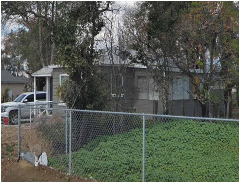
Plate 3.3-47: East façade of the 16172 Santa Ana Avenue building, facing northwest.
