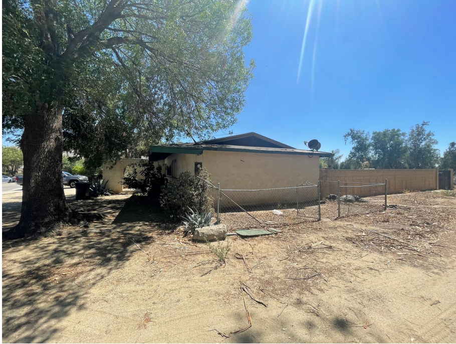
Plate 3.3–14: North façade of the 10818 Oleander Avenue building, facing south.
