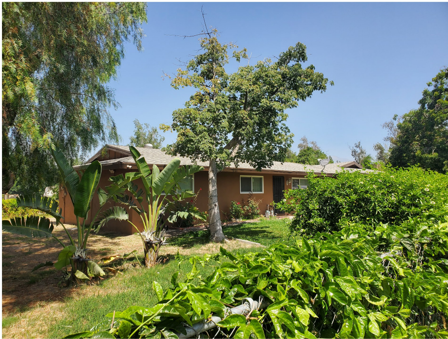
Plate 3.3–25: East façade of the 10888 Oleander Avenue building, facing northwest.
