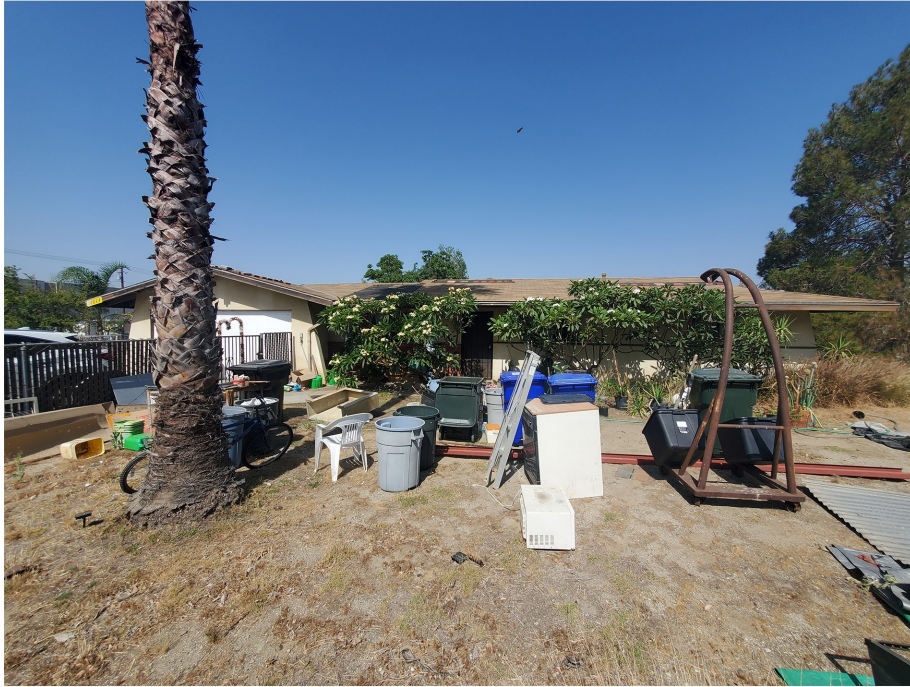
Plate 3.3–20: East façade of the 10864 Oleander Avenue building, facing west.
