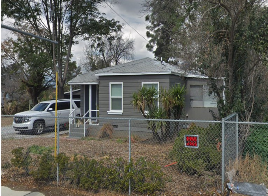
Plate 3.3-46: South façade of the 16172 Santa Ana Avenue building, facing northwest.
