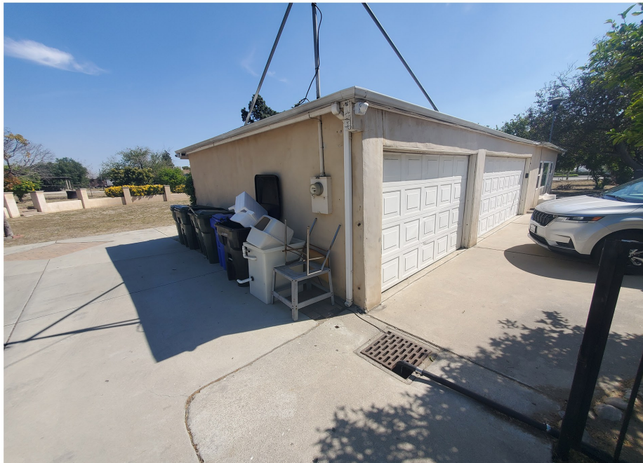
Plate 3.3-65: North (left) and west (right) façades of the 10861 Citrus Avenue garage addition, facing southeast.
