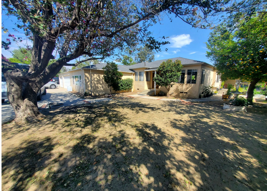
Plate 3.3–62: West (left) and south (right) façades of the 10861 Citrus Avenue building, facing northeast.
