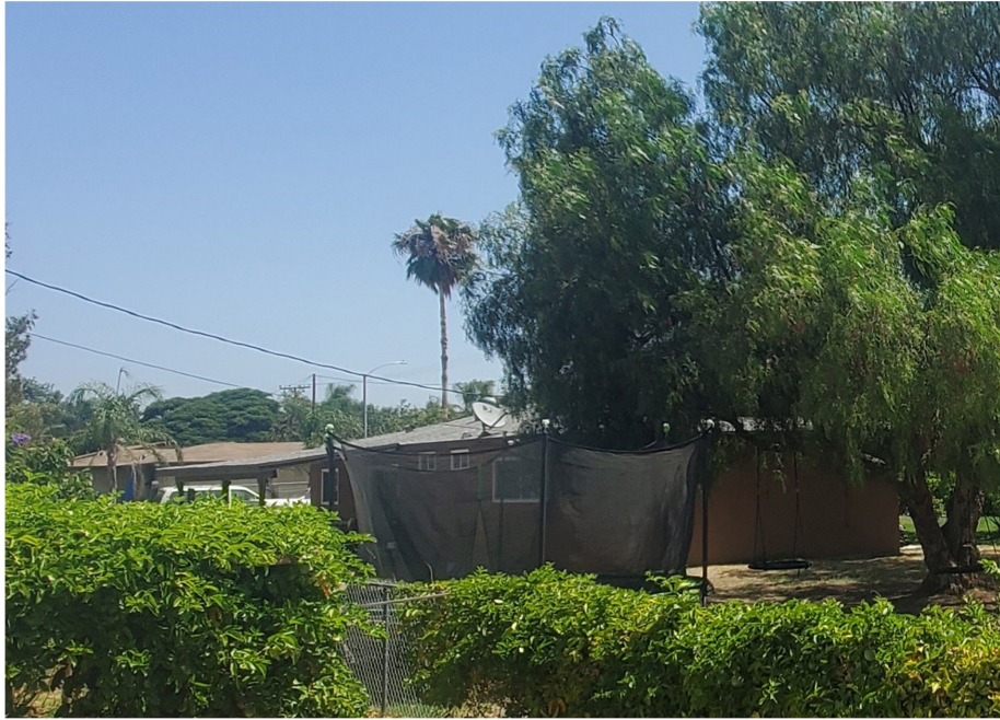
Plate 3.3–28: West façade of the 10888 Oleander Avenue building, facing northeast.
