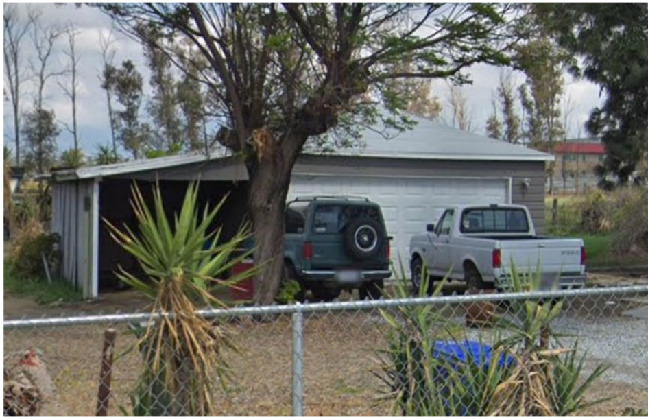
Plate 3.3–51: 2018 view of the 16172 Santa Ana Avenue detached garage, facing northeast.
