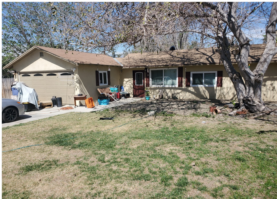
Plate 3.3–59: South façade of the 16228 Santa Ana Avenue building, facing northwest.
