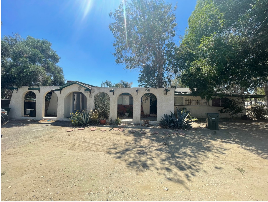
Plate 3.3-12: East façade of the 10818 Oleander Avenue building, facing west.
