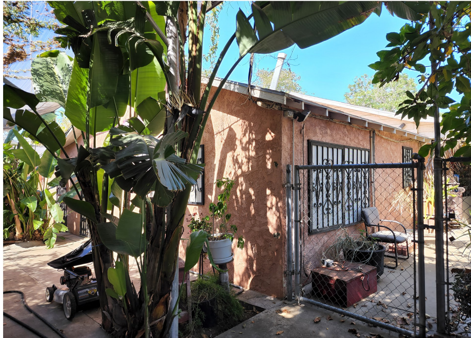
Plate 3.3-56: West (left) and south (right) façades of the 16204 Santa Ana Avenue building, facing northeast.
