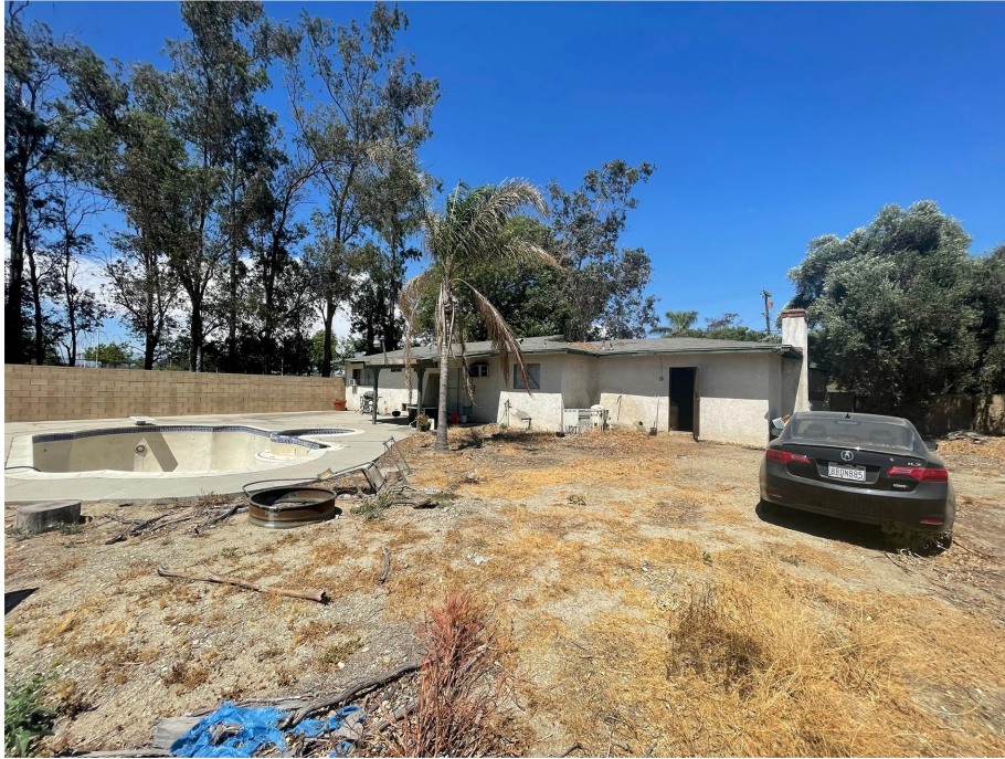
Plate 3.3-16: West façade of the 10818 Oleander Avenue building, facing east.
