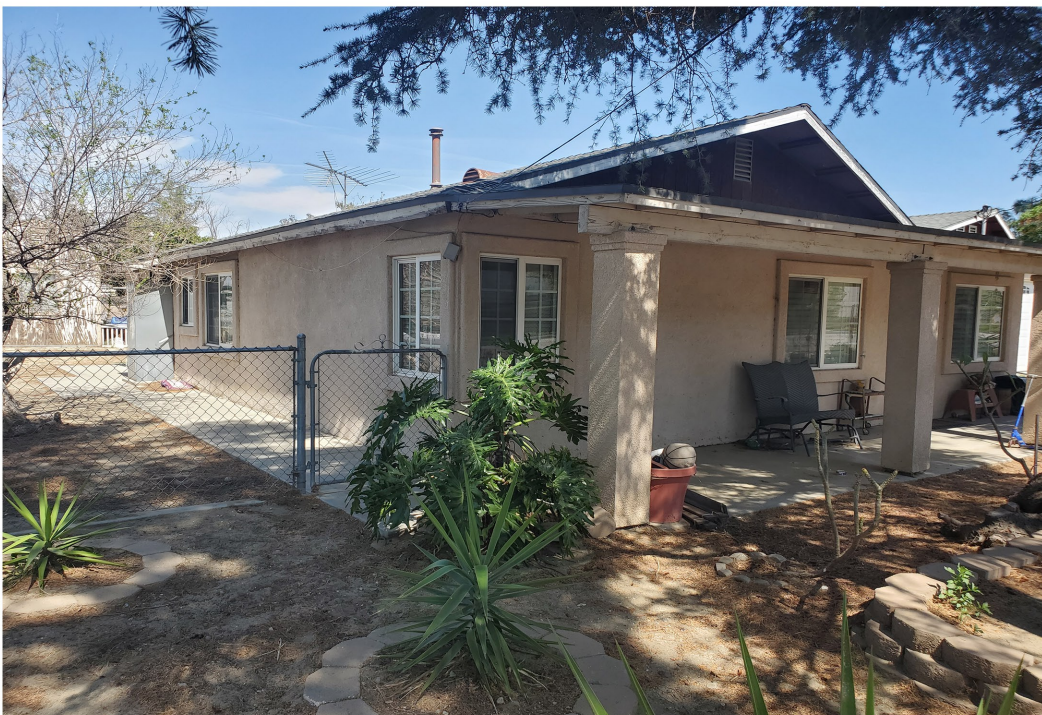
Plate 3.3-39: West (left) and south (right) façades of the 16156 Santa Ana Avenue building, facing northeast.
