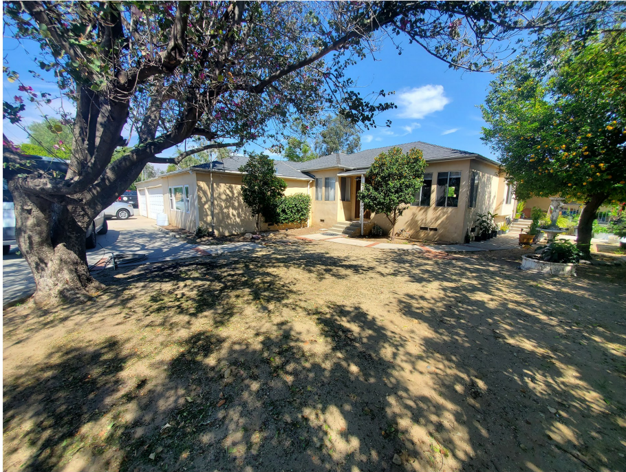
Plate 3.2-2: Overview of the project from the southwest corner, facing northeast.
