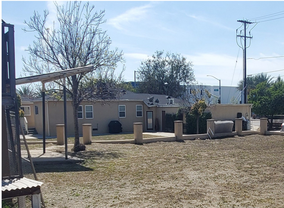
Plate 3.3-64: North façade of the 10861 Citrus Avenue building, facing southwest.
