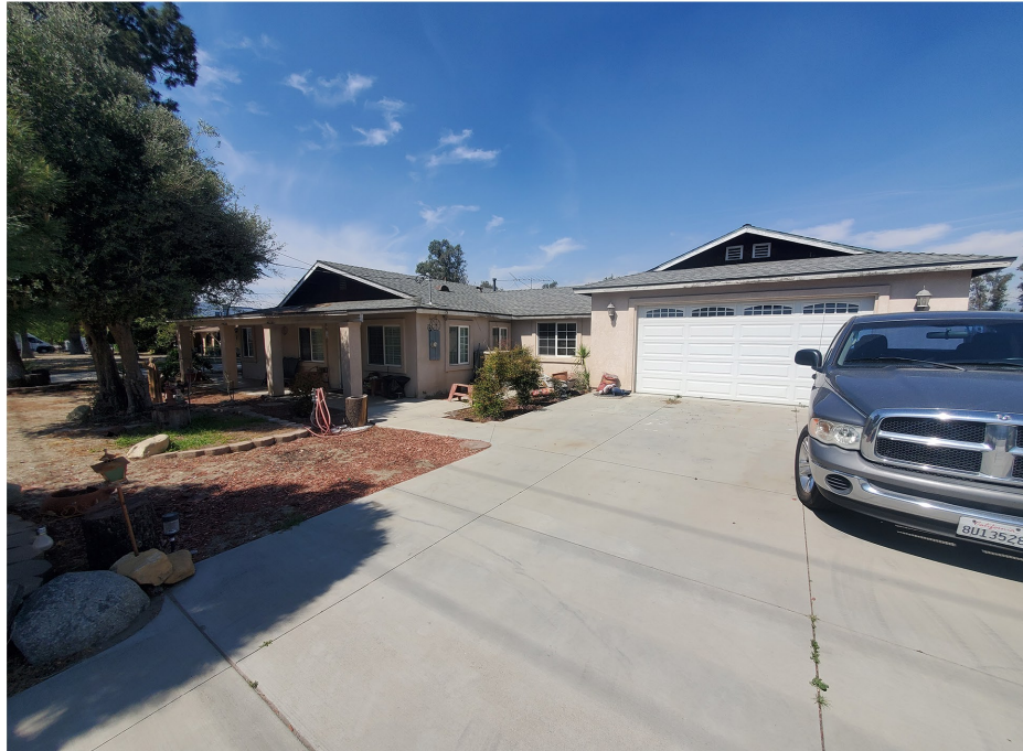
Plate 3.3–42: South façade of the 16156 Santa Ana Avenue building, facing northwest.
