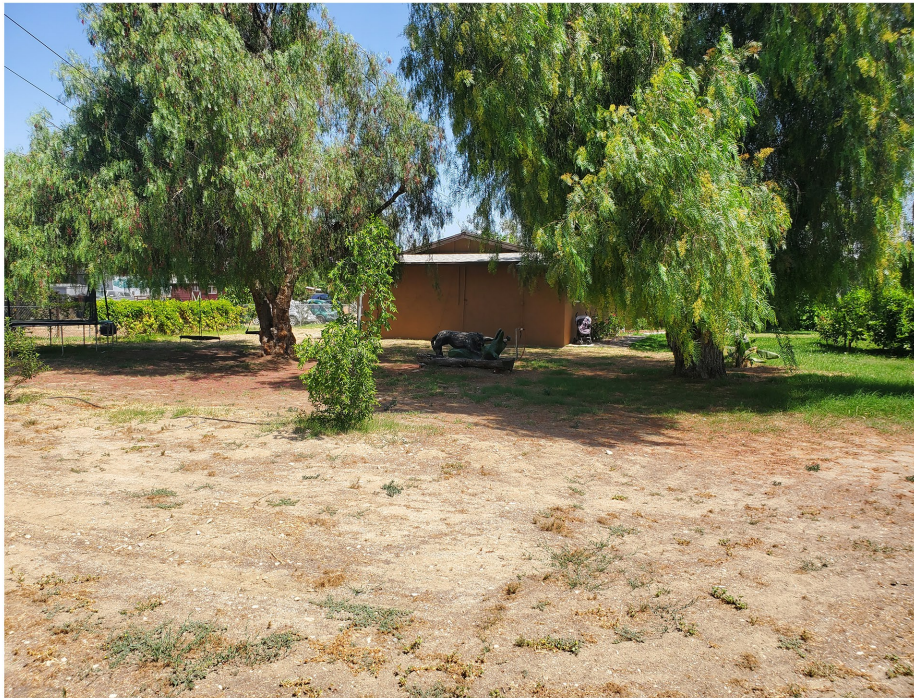
Plate 3.3–27: South façade of the 10888 Oleander Avenue building, facing north.
