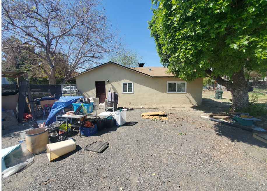
Plate 3.3–60: East façade of the 16228 Santa Ana Avenue building, facing west.
