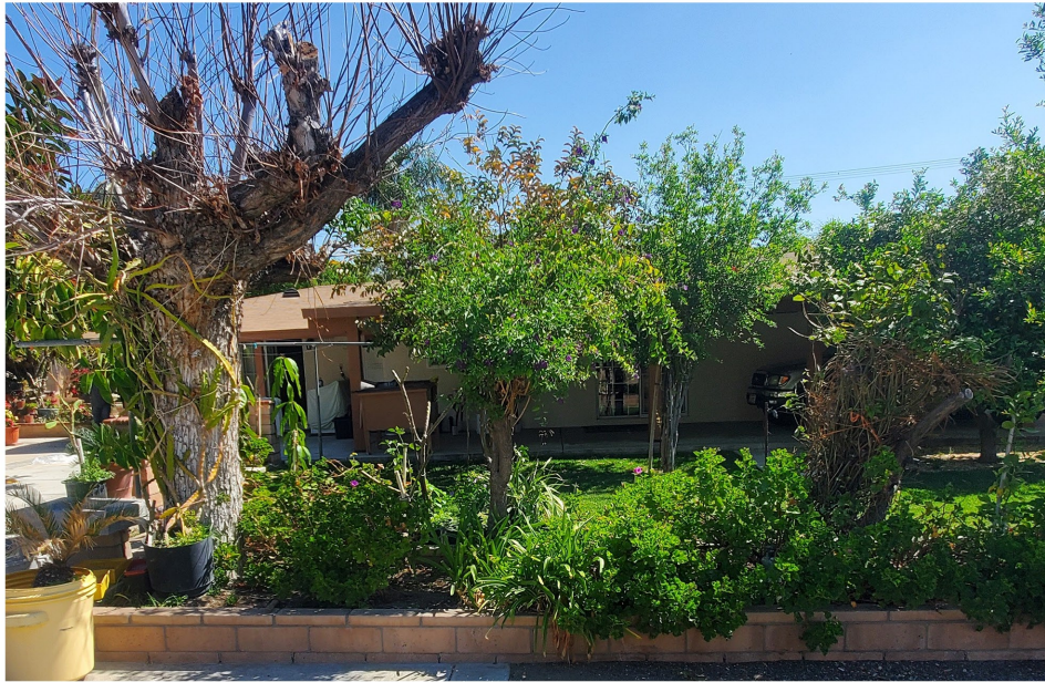
Plate 3.3-19: West façade of the 10840 Oleander Avenue building, facing east.
