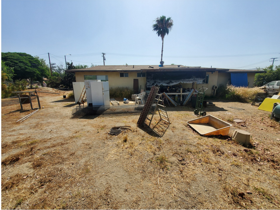
Plate 3.3–24: West façade of the 10864 Oleander Avenue building, facing east.
