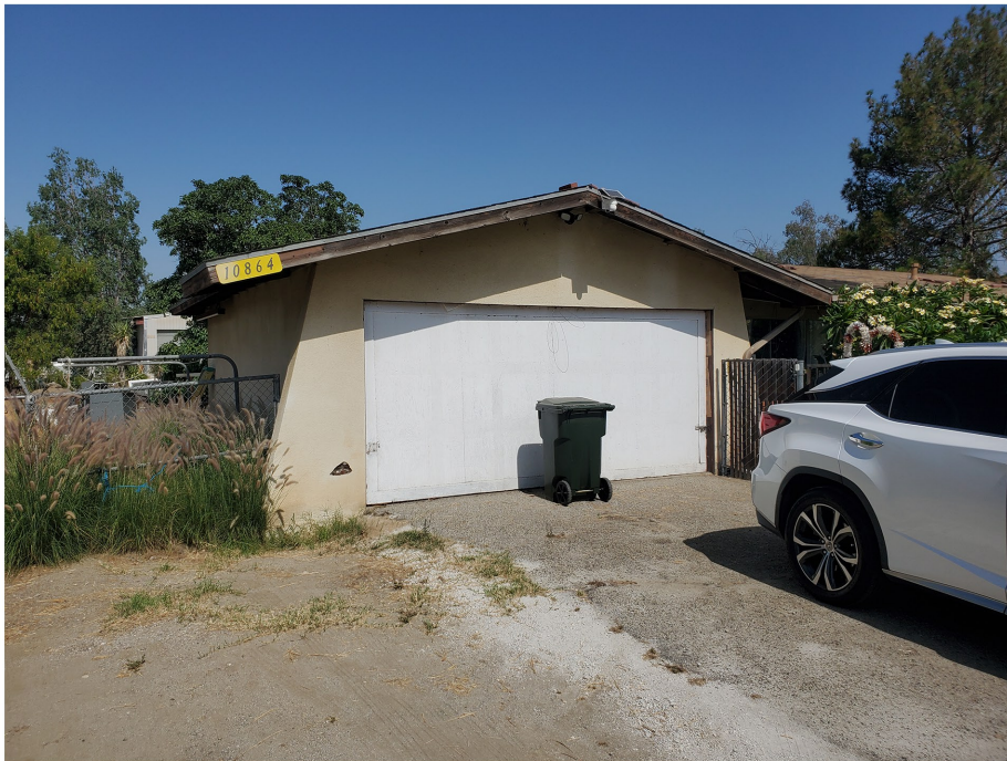
Plate 3.3–21: East façade of the 10864 Oleander Avenue attached garage, facing northwest.
