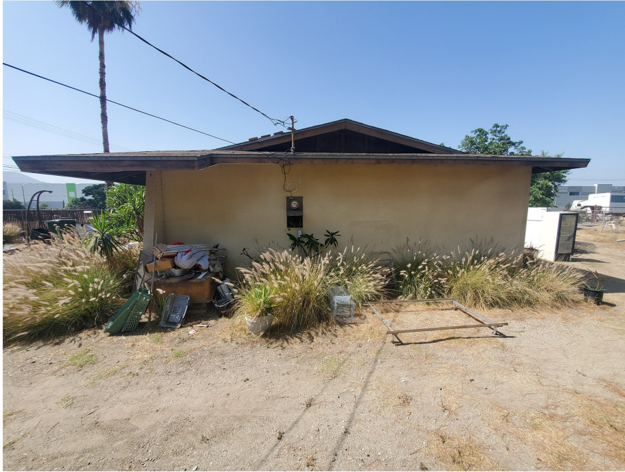
Plate 3.3–22: North façade of the 10864 Oleander Avenue building, facing south.
