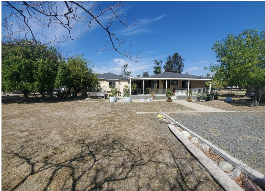
Plate 3.3–63: South Façade of the the 10861 Citrus Avenue building, facing north.
