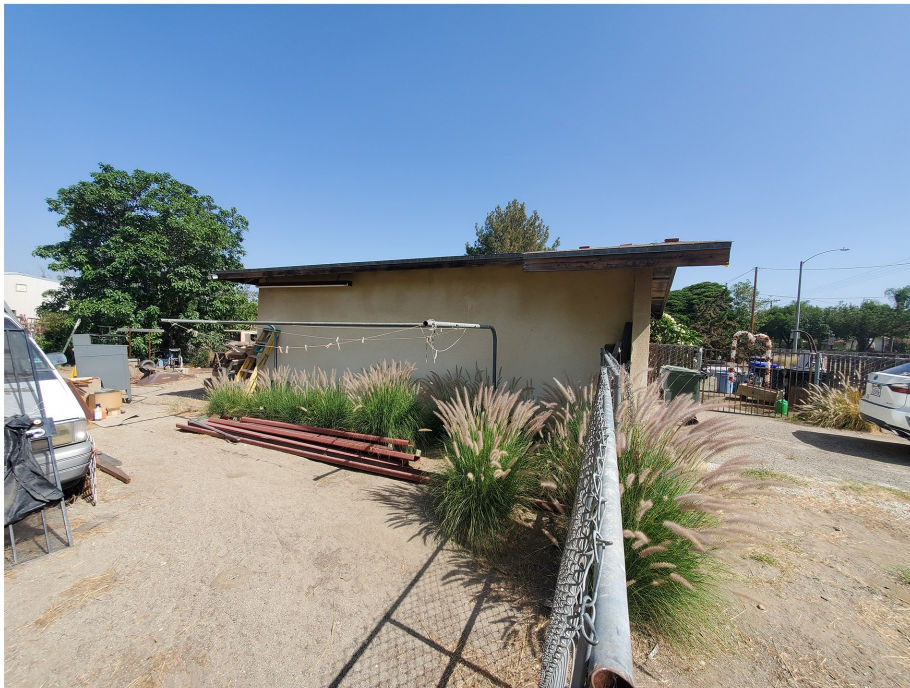
Plate 3.3–23: South façade of the 10864 Oleander Avenue attached garage, facing north.
