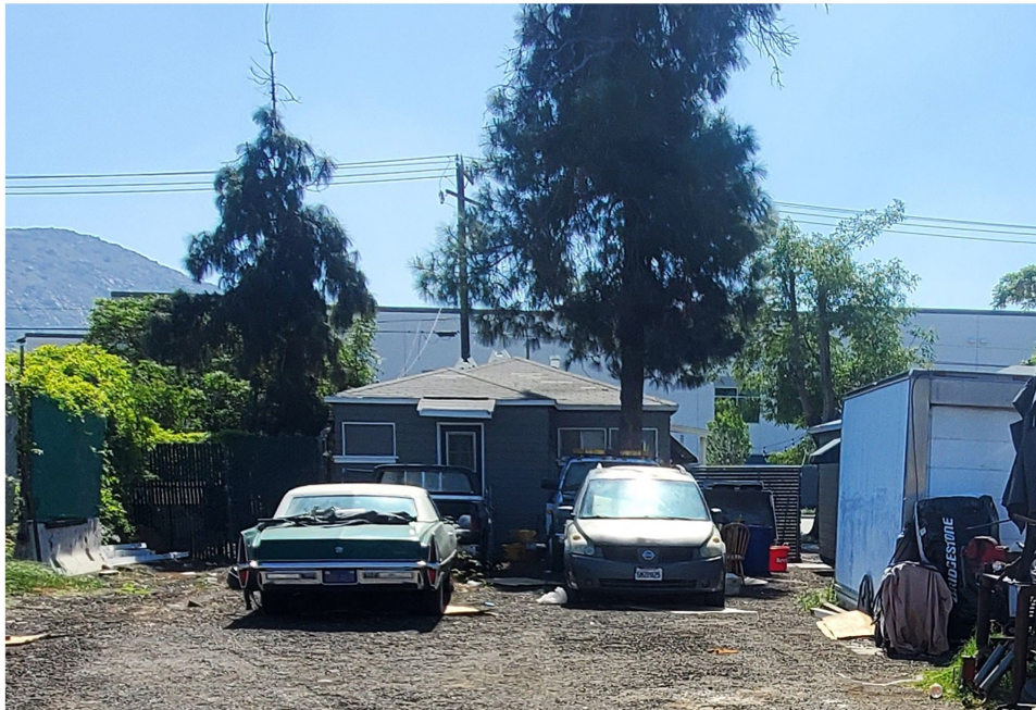
Plate 3.3–48: North façade of the 16172 Santa Ana Avenue building, facing south.
