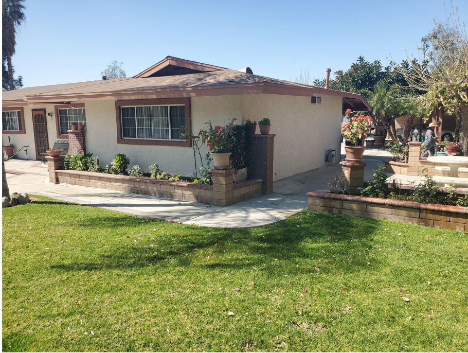
Plate 3.3-18: East (left) and north (right) façades of the 10840 Oleander Avenue building, facing southwest.
