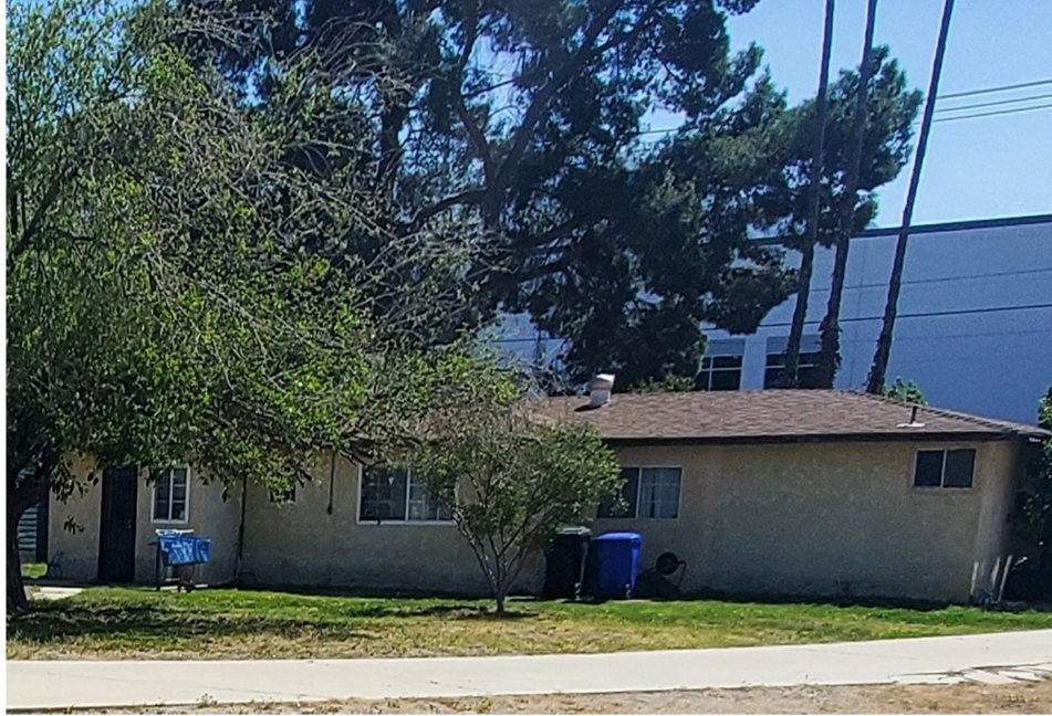
Plate 3.3-30: North façade of the 16140 Santa Ana Avenue single-family residence, facing southwest.
