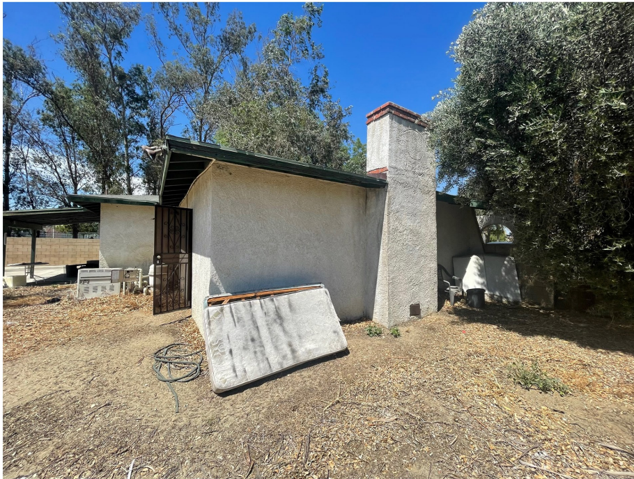
Plate 3.3–15: South façade of the 10818 Oleander Avenue building, facing north.
