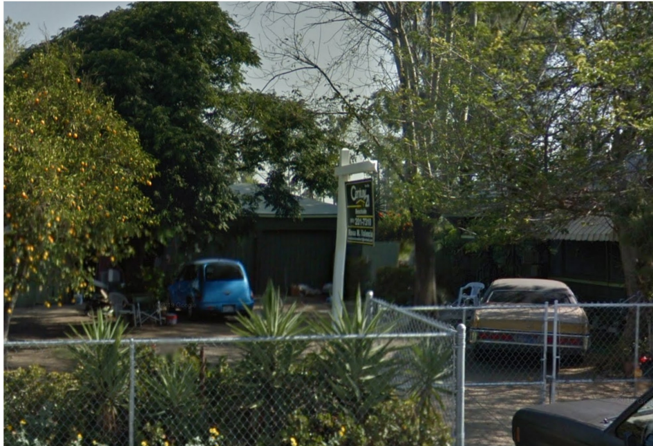
Plate 3.3–50: 2015 view of the 16172 Santa Ana Avenue detached garage, facing northeast.
