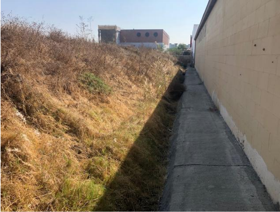
Photograph 5. Photo showing the concrete-lined v-ditch on the southern parcel border. Ground squirrel and desert cottontail individuals and burrows were observed on the slope.
