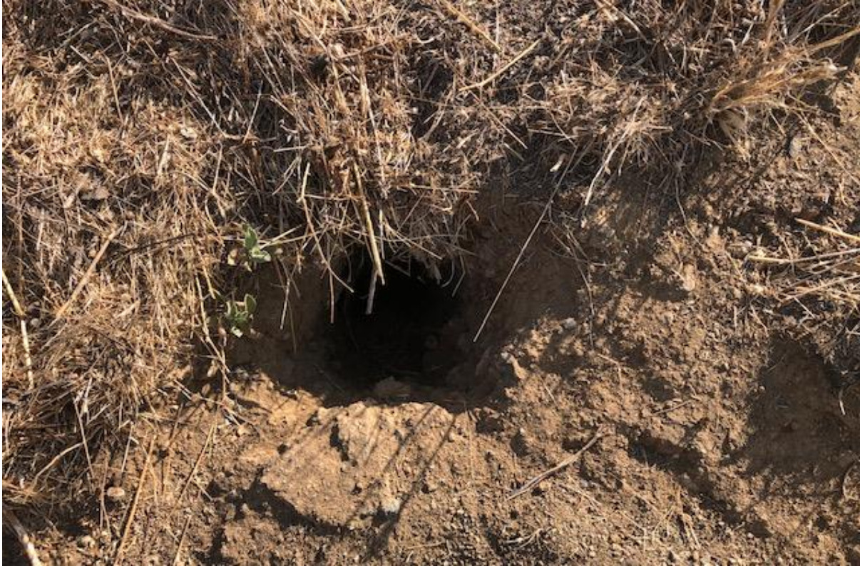
Figure 6 Southwest Portion of Project Site, Close Up View of Burrow and Exposed Soils
