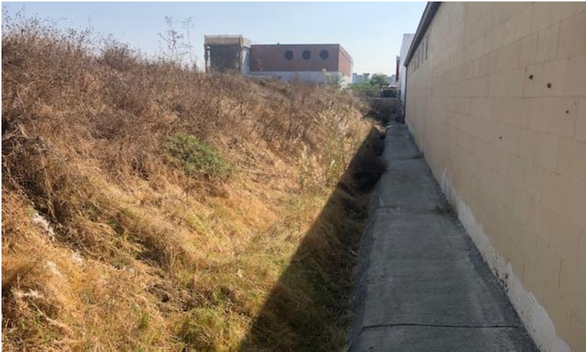
Figure 7 Southern Edge of Project Site, View Southwest
