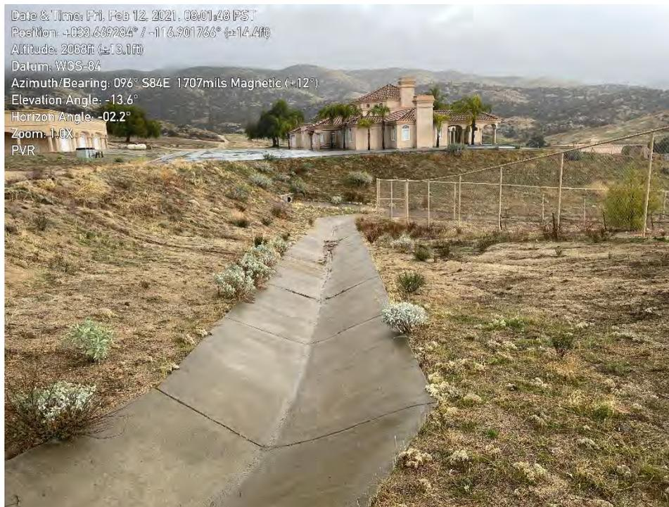
**PHOTOGRAPH 11:** The concrete V-ditch of Feature A<sub>3</sub>.
